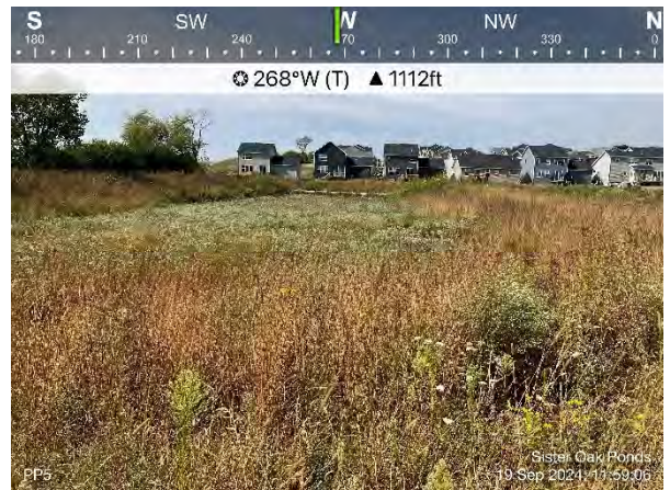
Photo #10 Photo point 5, view west toward the infiltration basin and the berm between the basin and wet pond
