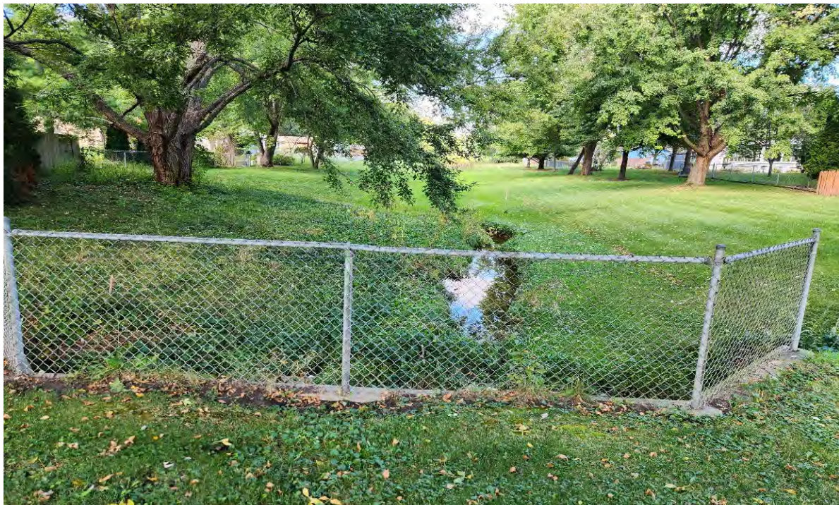
Figure 2. The grassed waterway looking upstream of Buckeye Road. This segment of channel is relatively stable, but this photo shows channel incision beginning at the downstream end of the reach (photo Inter-Fluve).
