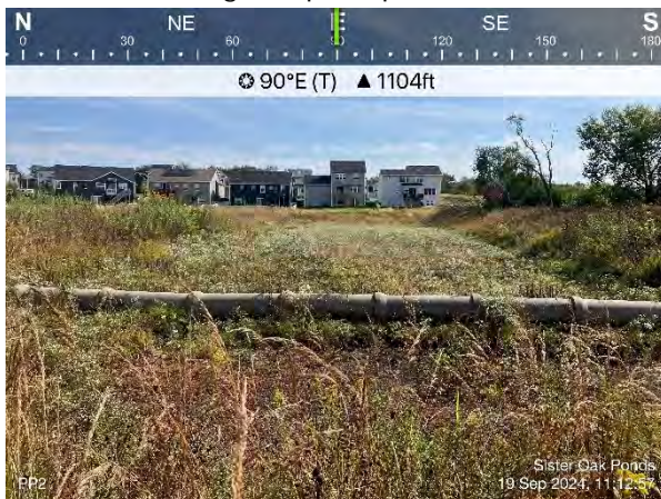
Photo #5 Photo point 2, view east towards the infiltration basin
