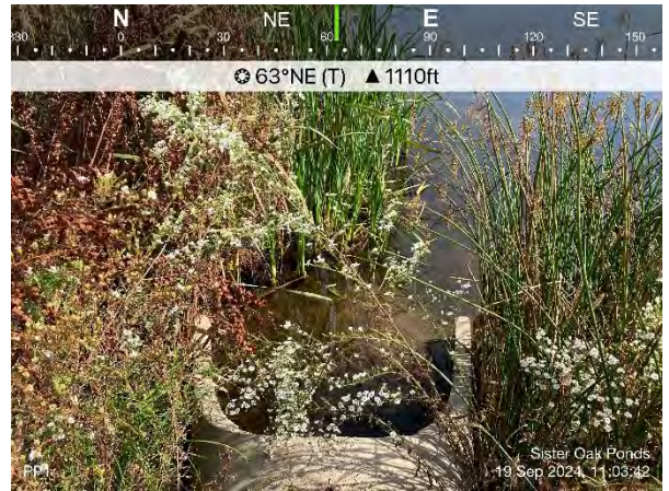
Photo #2 Photo point 1, culvert at west side of wet pond
