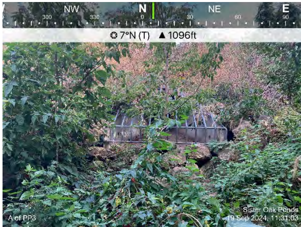
Photo #7 Photo point 3, view north towards tree saplings growing in riprap below infiltration basin culvert
