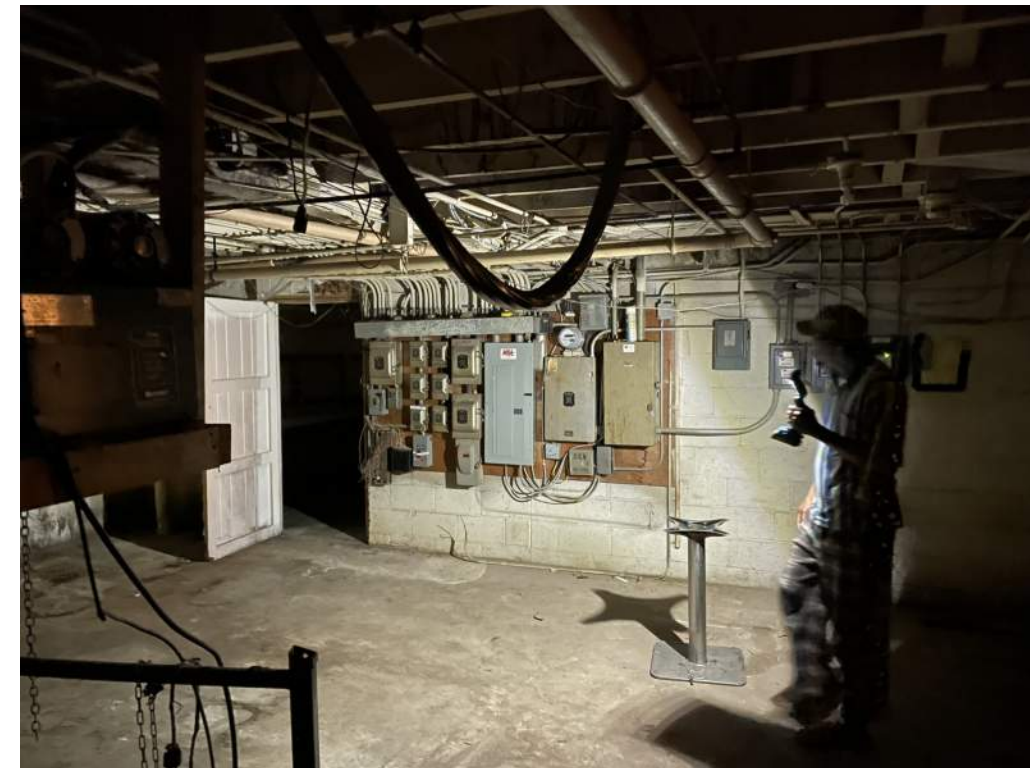
INTERIOR VIEW BASEMENT SPACE
