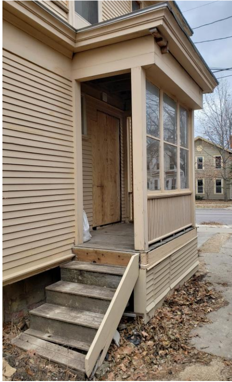
Rear Porch lkg NW
