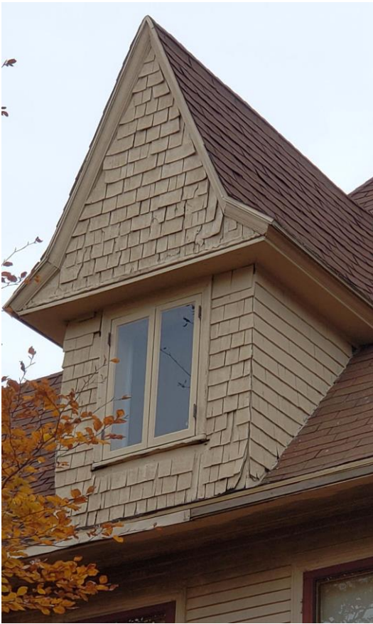
Spaight-side dormer sheathing repairs
