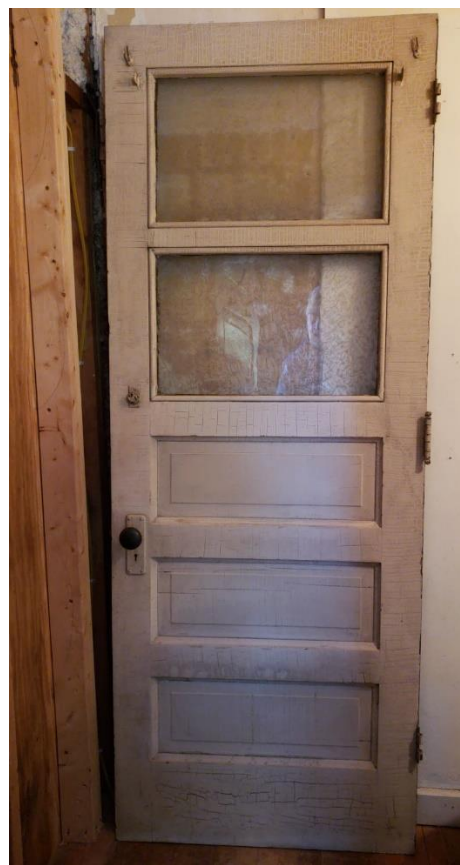
Rear porch door/window reinstall
