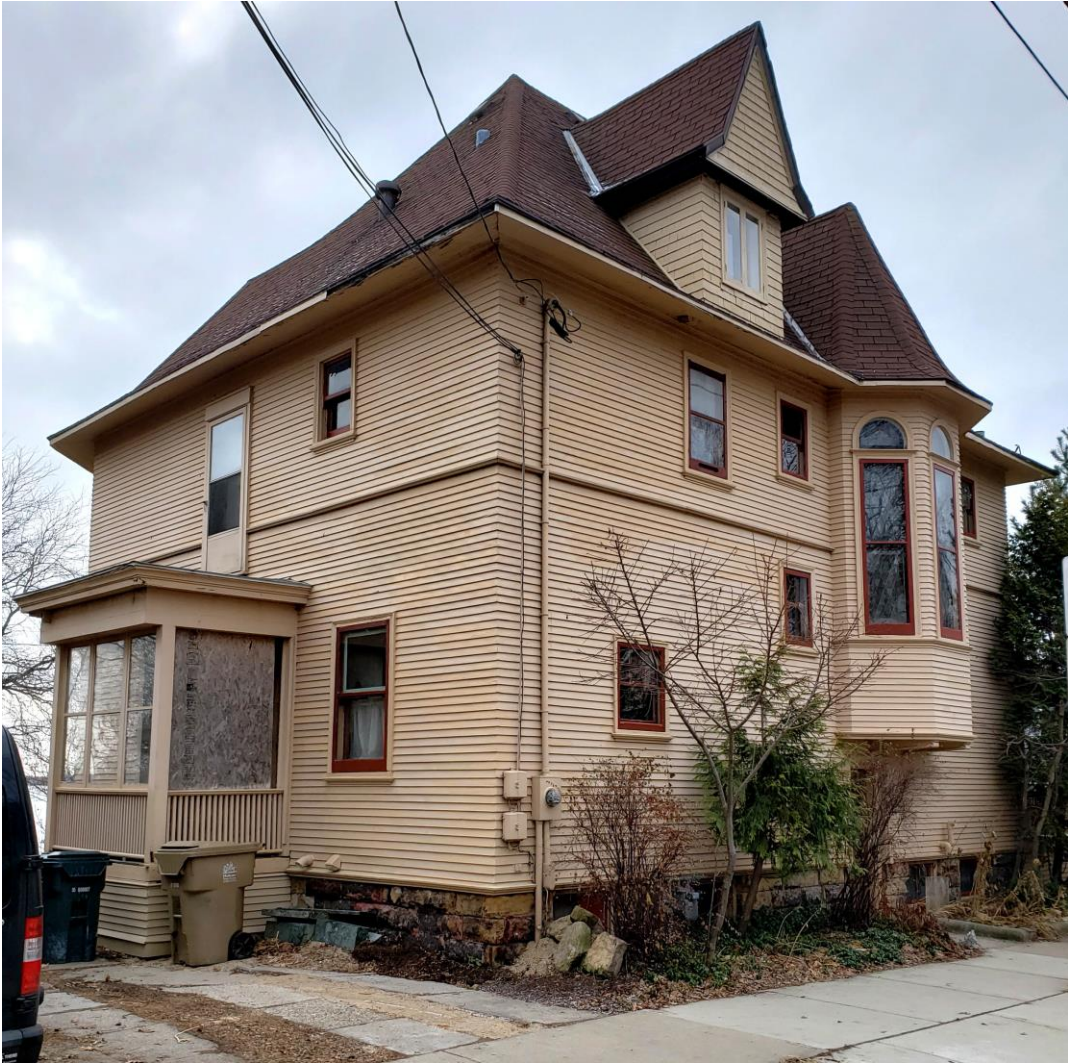
Rear Porch lkg S along Jenifer
