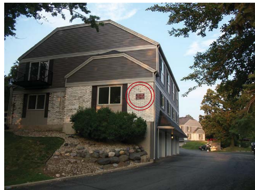
REPRESENTATIVE SAMPLE OF BUILDING ID SIGN BEING REPLACED
