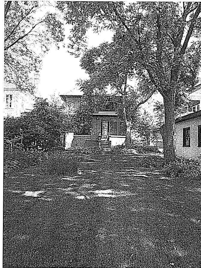
EXISTING RESIDENCE - WEST ELEVATION
