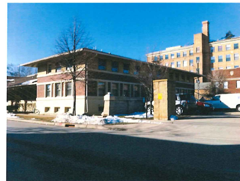
ADJACENT BUILDING ON E MIFFLIN STREET
