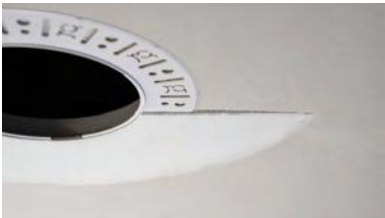
Partially finished mud ring, showing cross-section detail.
