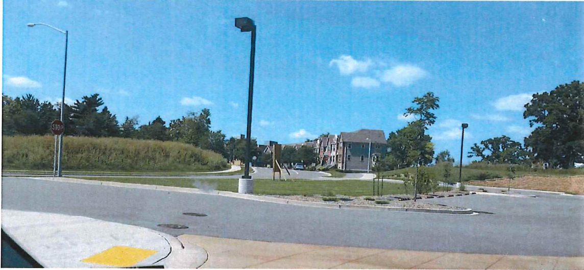
Existing site lighting and landscaping installed.
