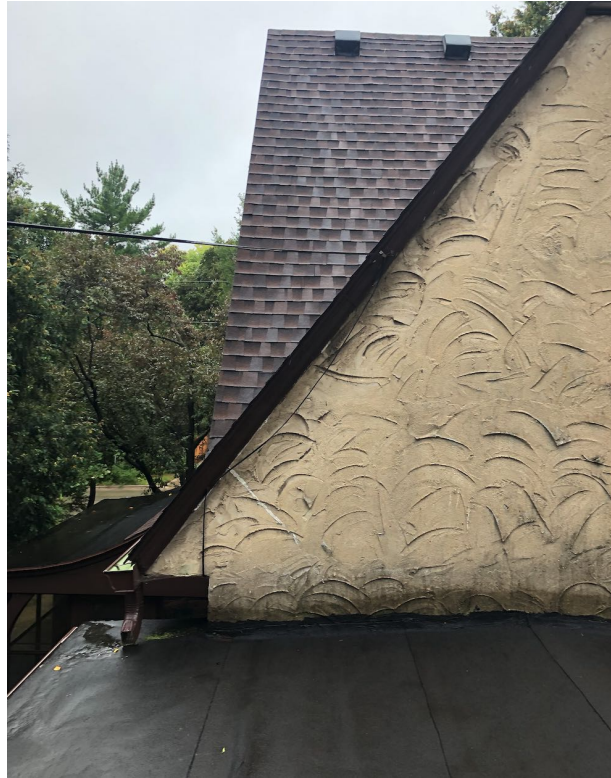
EXISTING MEMBRANE ROOF ABOVE SINGLE STORY FLAT ROOF STRUCTURE.
