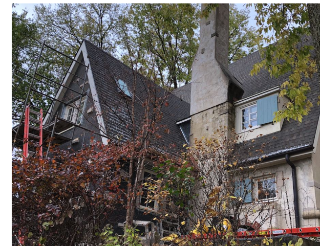
2114 VAN HISE AVE- IS A SIMILAR PROJECT TYPE THAT WE RECENTLY SECURED LANDMARKS APPROVAL FOR. HERE A MASTER BATHROOM WITH STEEP PITCH IS INTEGRATED WITH SHED DORMERS ON THE MAIN ROF.
