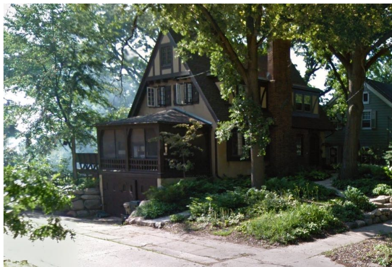
114 BASCOM PL - DEMONSTRATES SHED DORMER ON STEEP SLOPE OF SECOND LEVEL ROOF TO PROVIDE HABITABLE SPACE UNDER THE ROOFLINE
