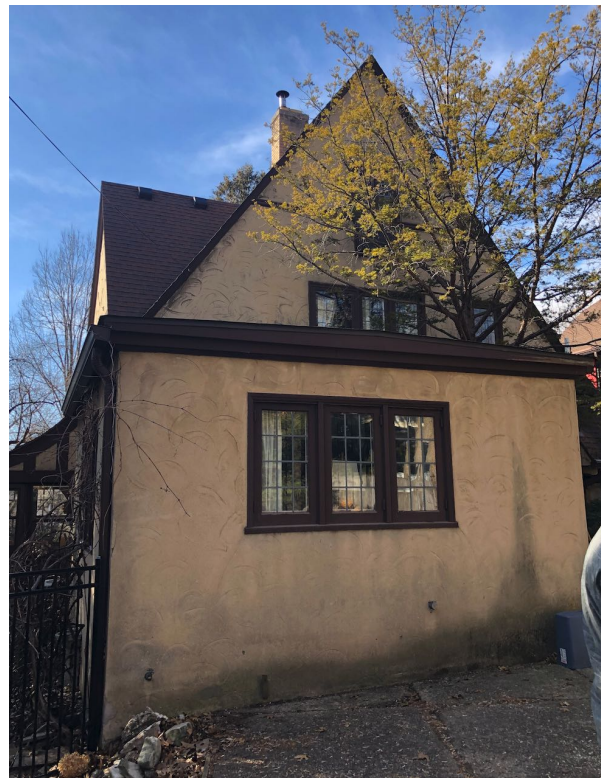
THIS PERSPECTIVE HINTS AT THE FORM OF THE SECOND LEVEL BATHROOM ADDITON ABOVE THE FLAT ROOF STRUCTURE
