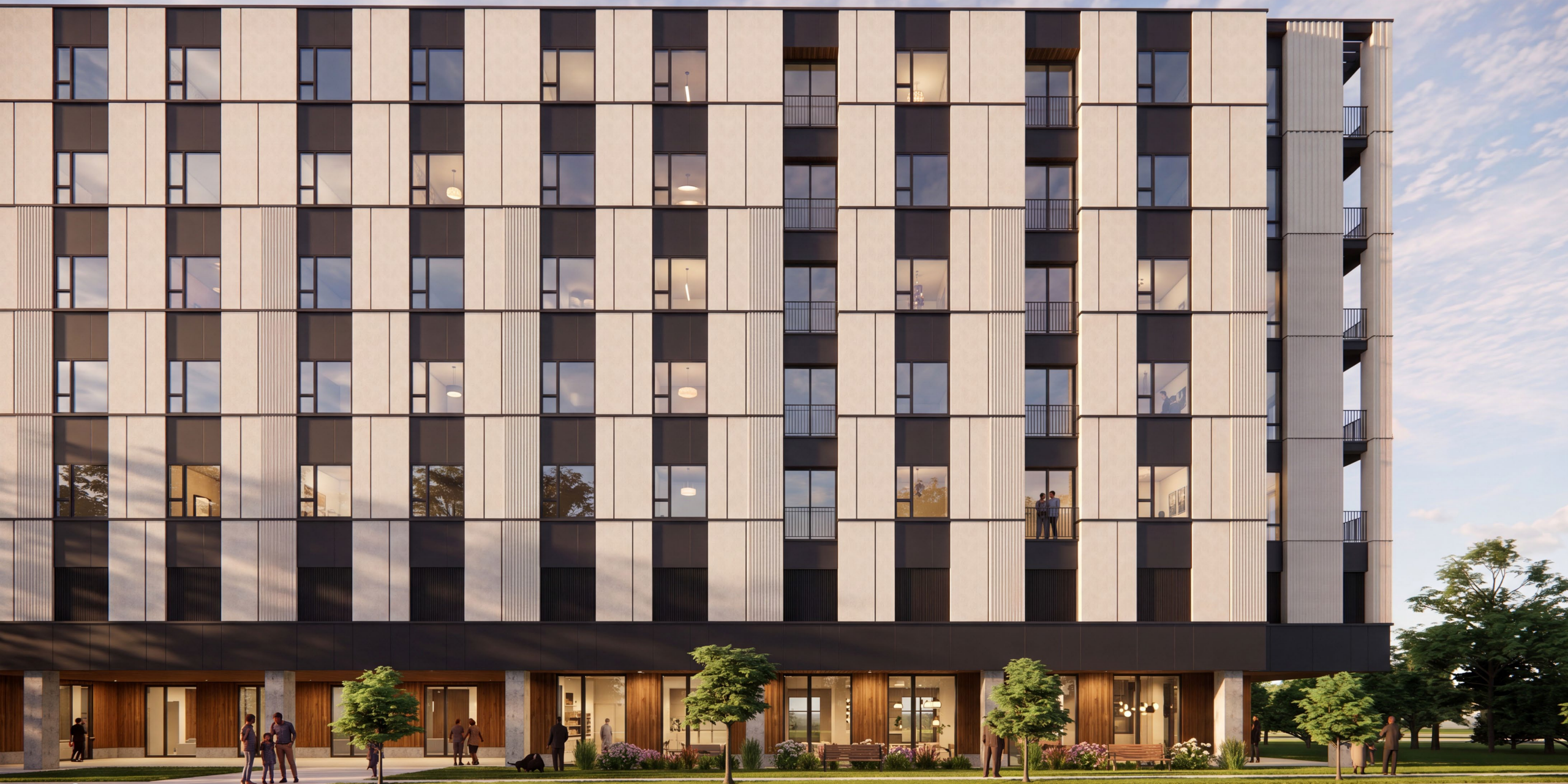
East Olin Ave – Façade Detail
