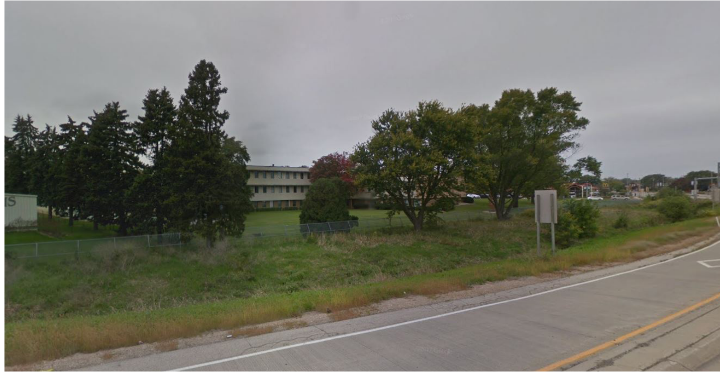
View from Hwy-12 West on-ramp
