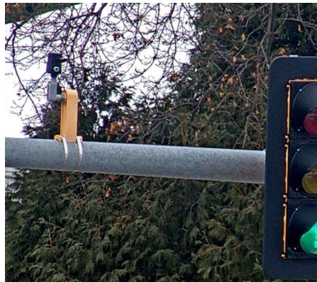
Emergency Vehicle Detector (EVD) on Midvale and Mineral Point Rd.
