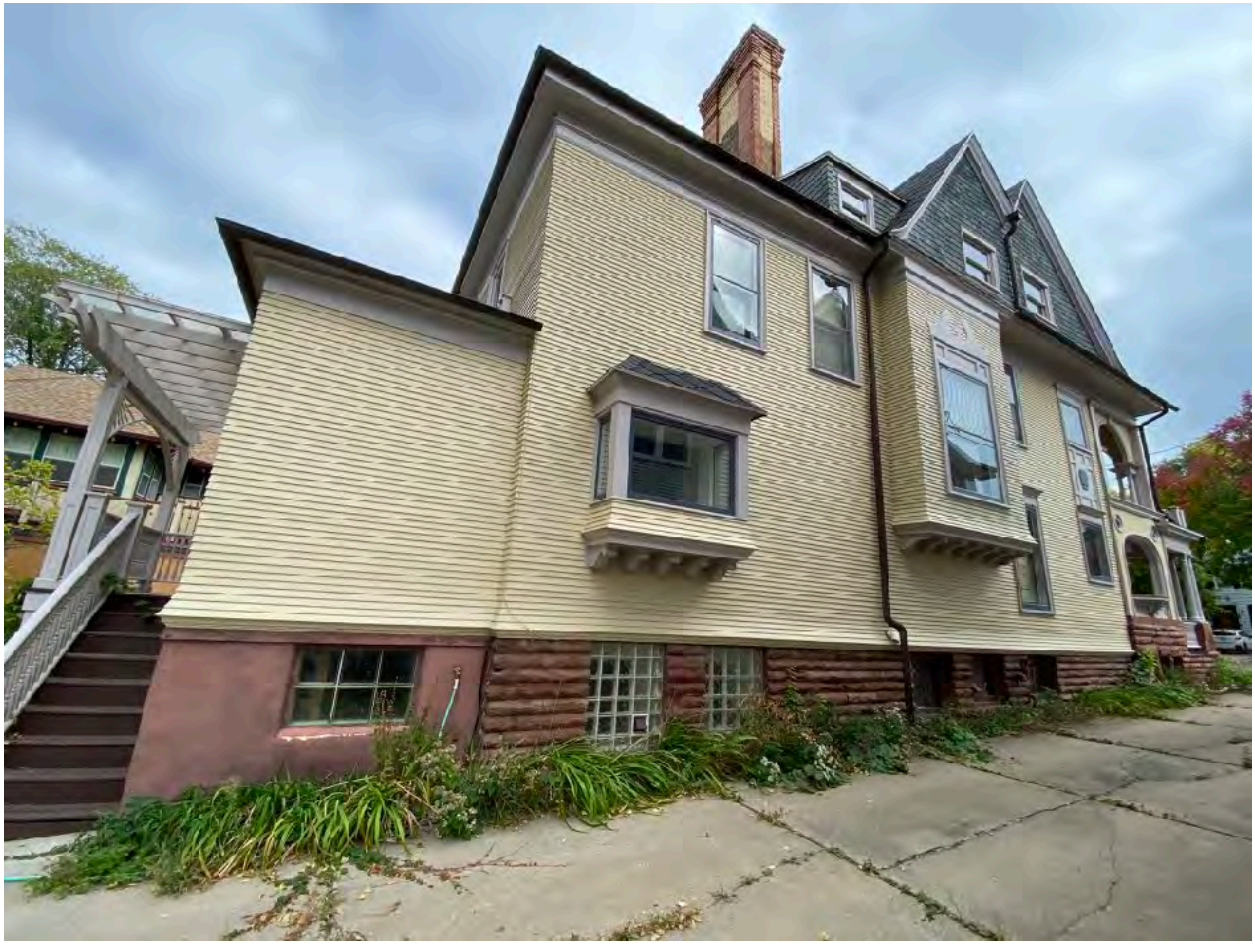
West Facing Elevation of 848 Jenifer Street
