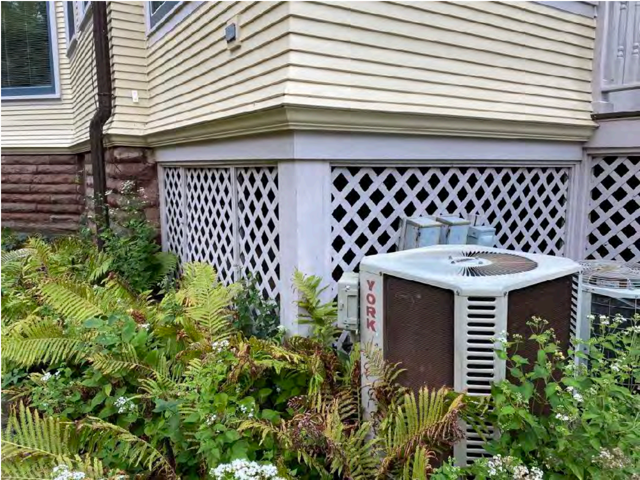
Photo of Non-Original Lattice Enclosure
