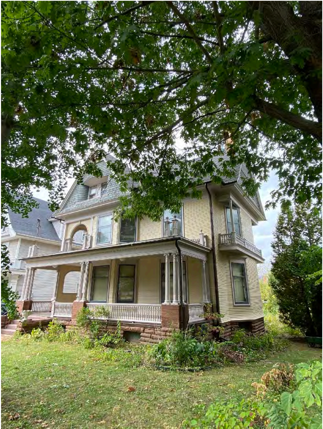
South/East Facing Elevation of 848 Jenifer Street
