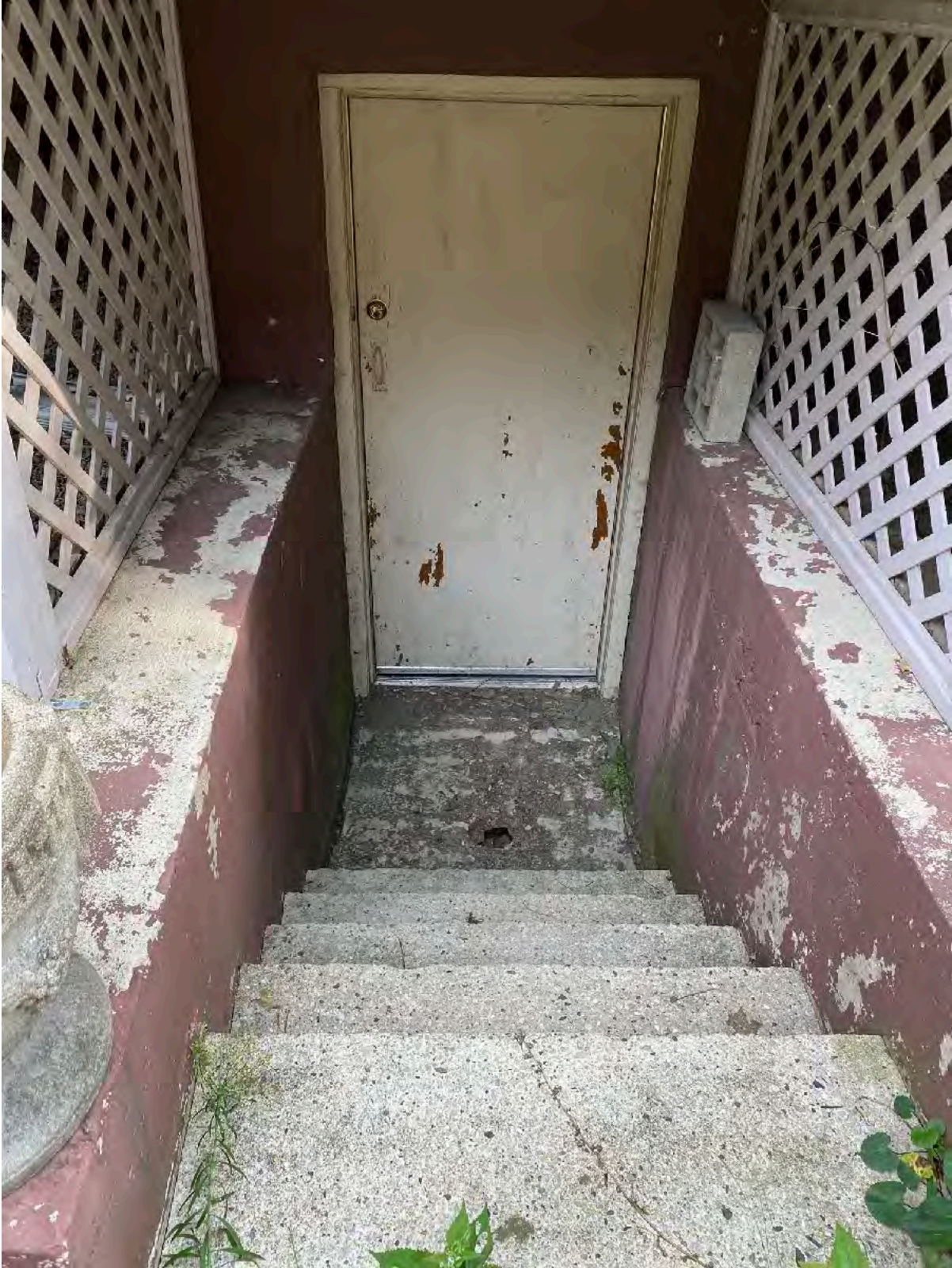
Photo of Existing Lower Level Entry
