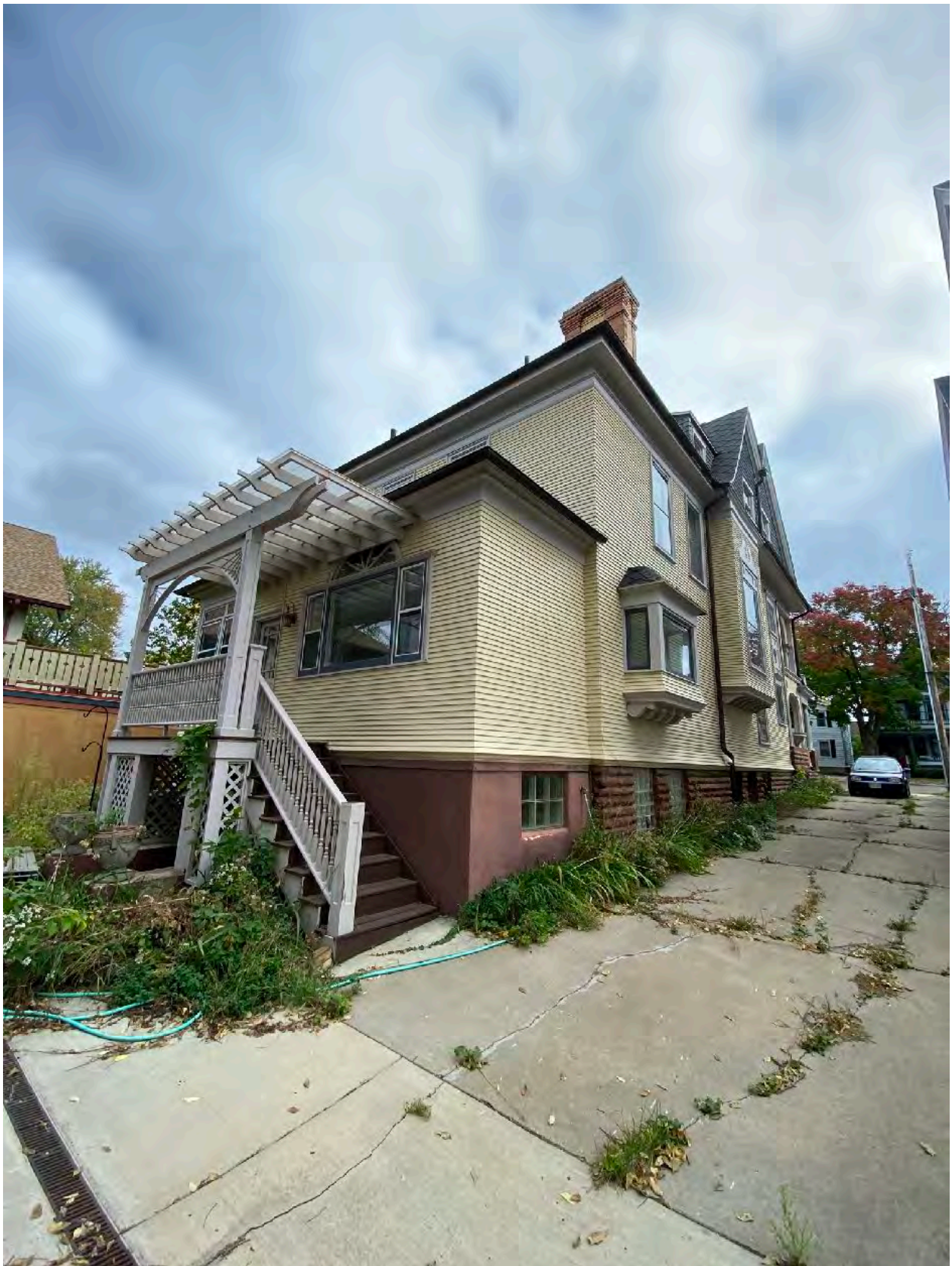
North/West Facing elevation of 848 Jenifer Street
