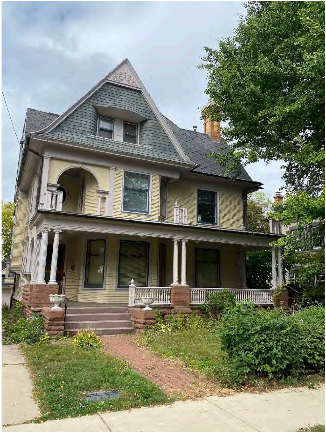
South Facing Elevation of 848 Jenifer Street
