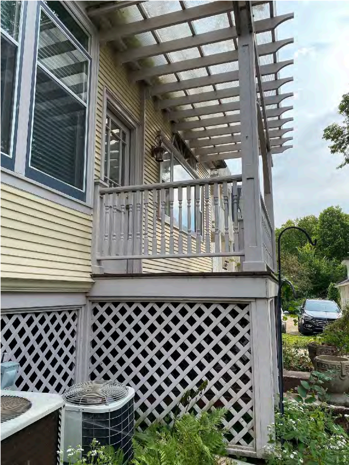
Photo of First Floor Entrance Door
