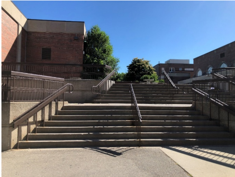
View of stairs to Plaza that are to be removed for addition.
