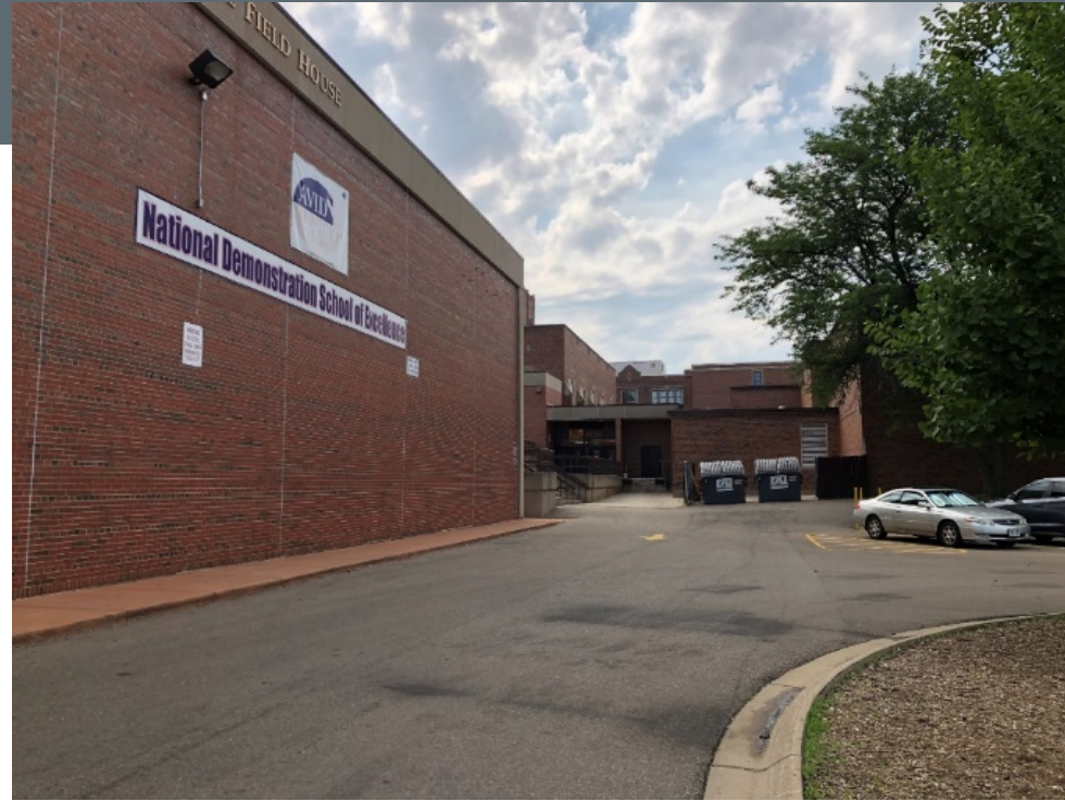
View of Addition location from parking lot, Fieldhouse on left.
