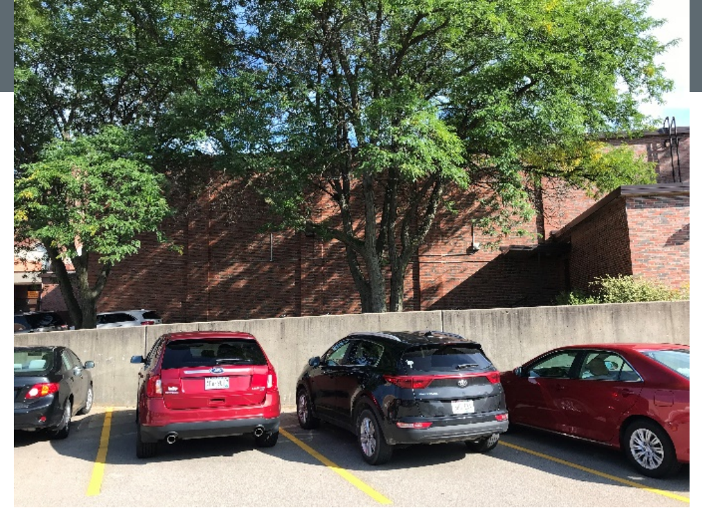
Standing in parking lot, looking at the west wall of pool.
