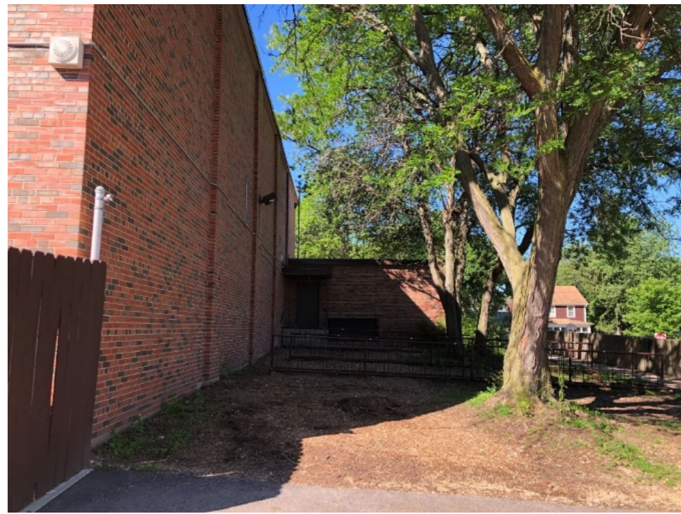
Standing at site of addition looking along west side of pool.
