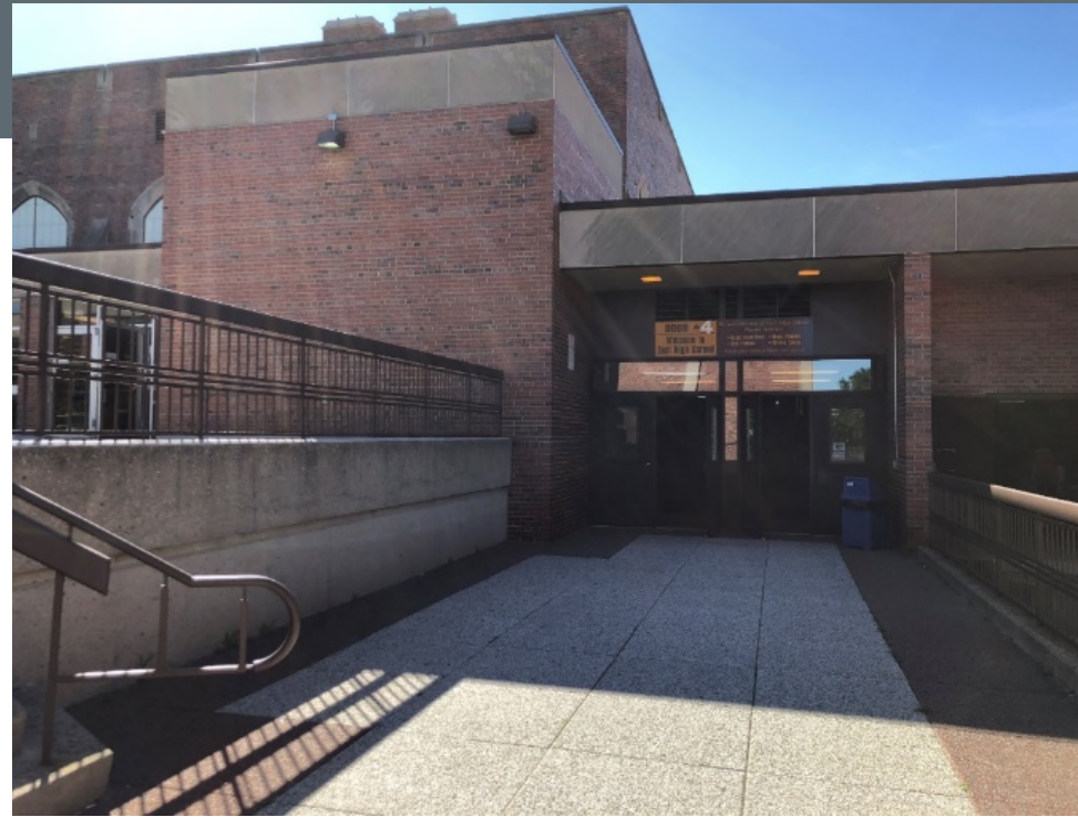
View of existing entrance that will remain, this will be the location of the new ramp from ground floor.
