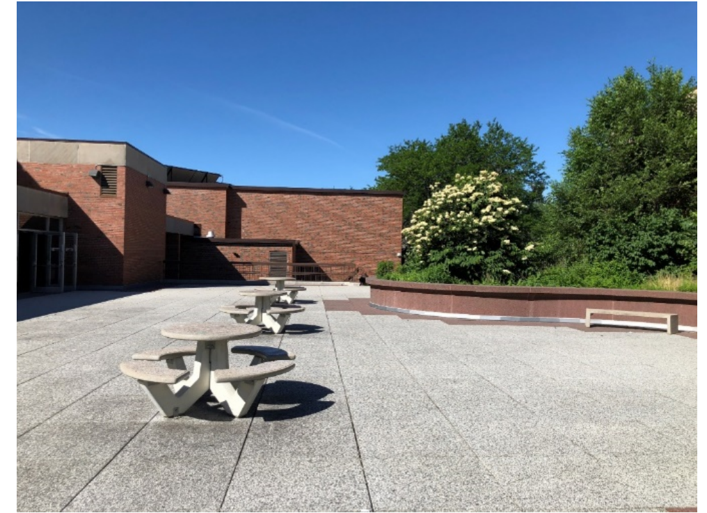
Standing on Plaza looking at site of addition, pool wall in the background.
