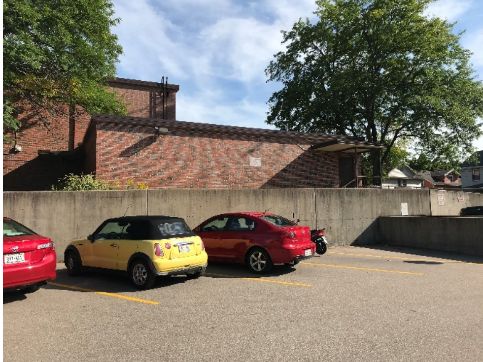
Standing in parking lot, looking south of pool.
