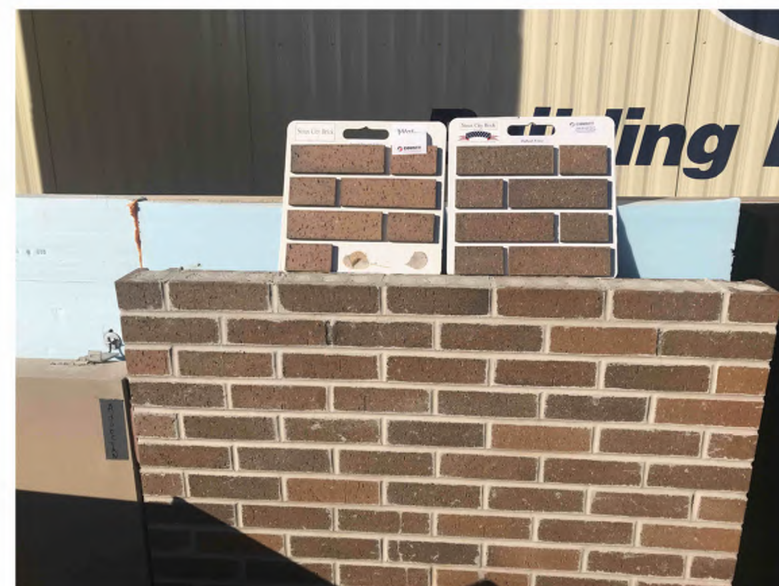
BRICK VENEER, COLOR SHALL BE SIOUX CITY, TOASTED FINE ART VELOUR, MODULAR
