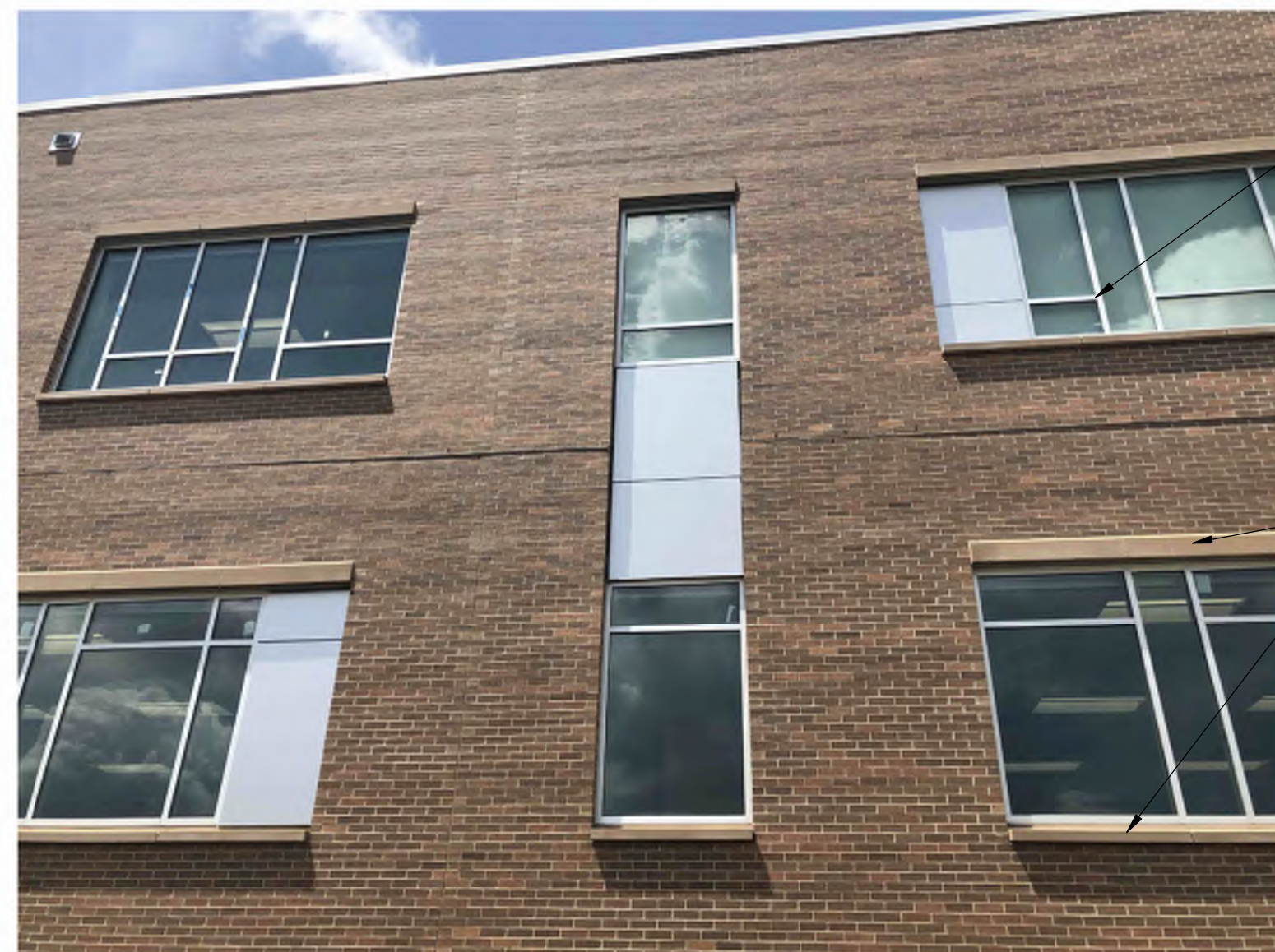
ALUMINUM STOREFRONT, COLOR SHALL BE CLEAR ANODIZED AS MANUFACTURED BY KAWNEER
