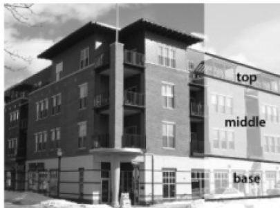
Figure D7: Building Articulation
