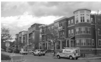
Figure D6: Building Alignment
