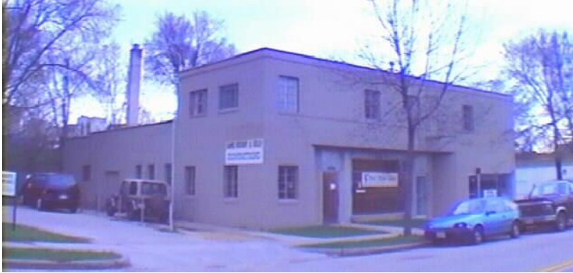
2544 University Ave: Commercial, unknown date of construction
