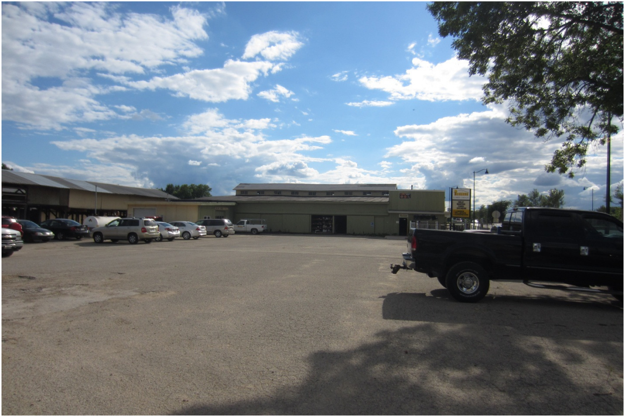
EXISTING DRIVEWAY, LOOKING SOUTH
