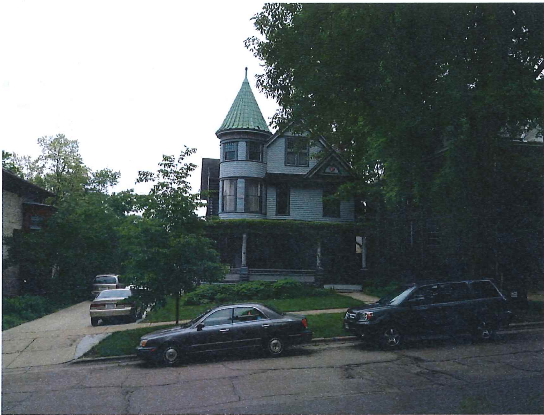
Residential building, across the street to the east
