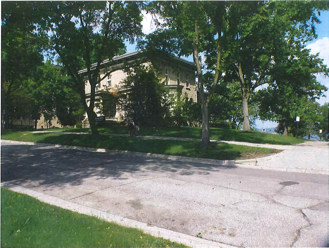
Front elevation from north
