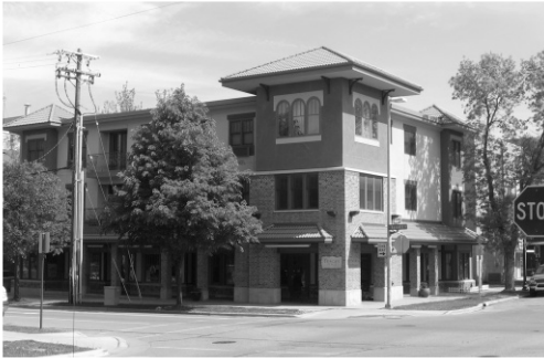
Figure D1: Entrance Orientation
