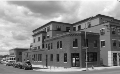
Figure D4: Variation in Roof Lines
