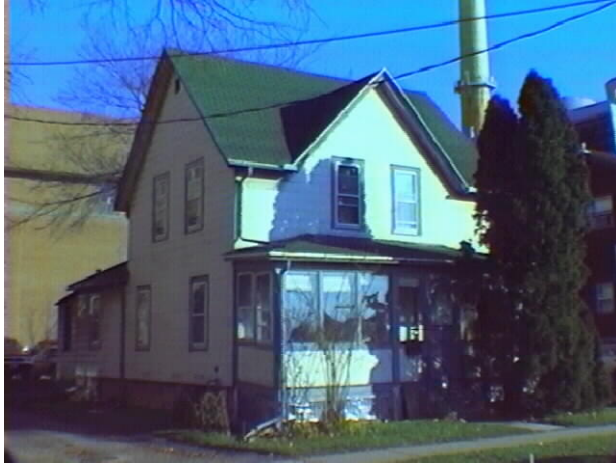
1208 Spring Street (1880 building)
