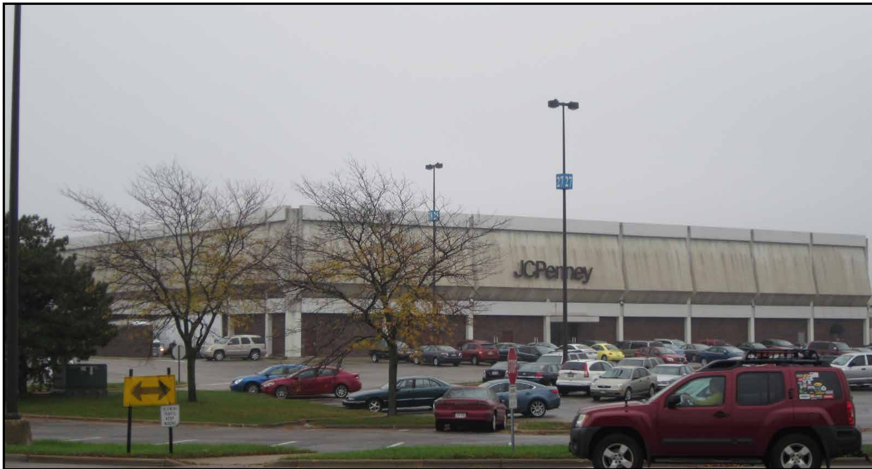
Adjacent Property to Southeast
