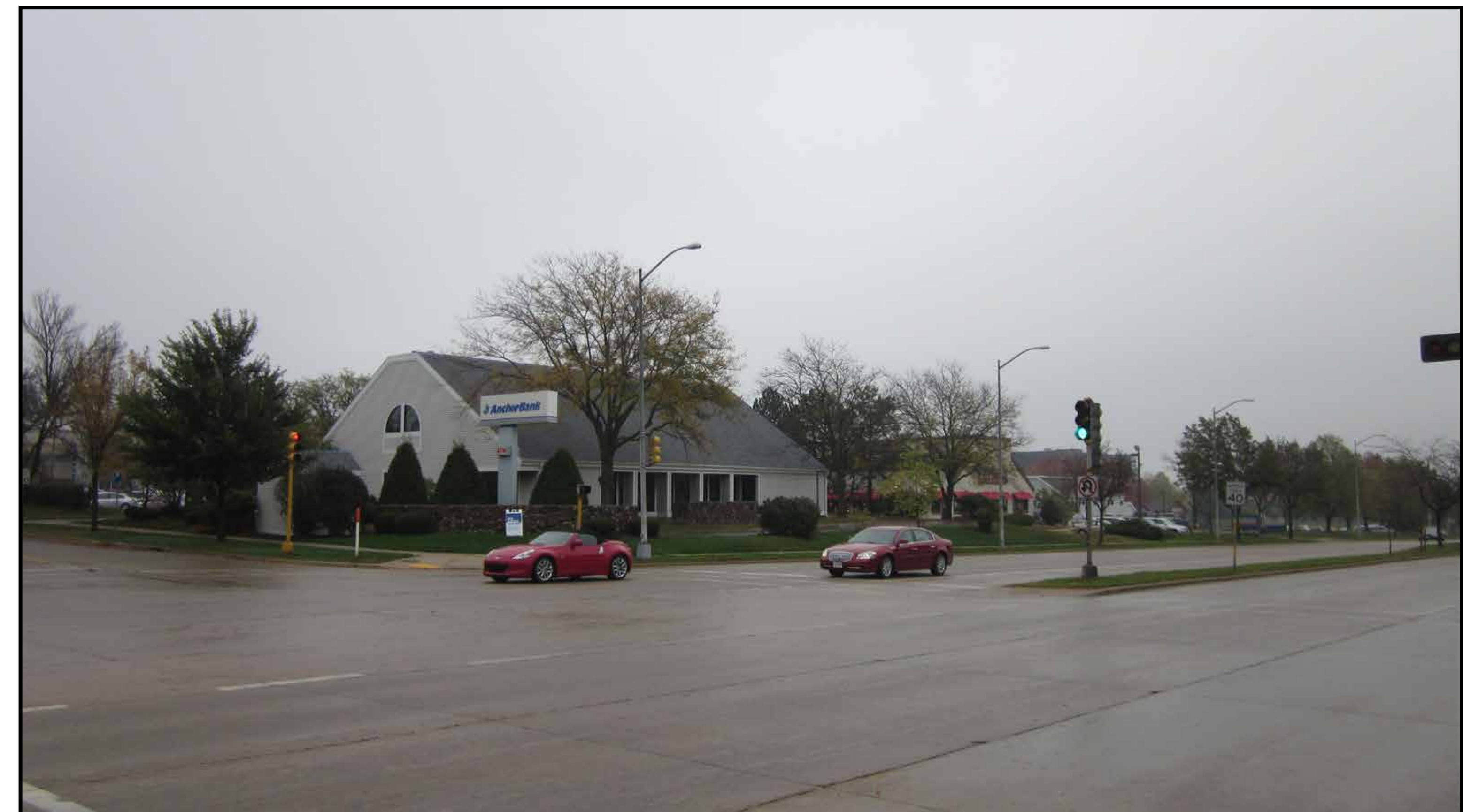
S. Westfield Road Intersection
