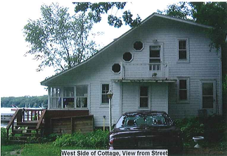
West Side of Cottage, View from Street
