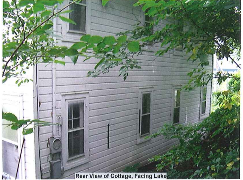
Rear View of Cottage, Facing Lake
