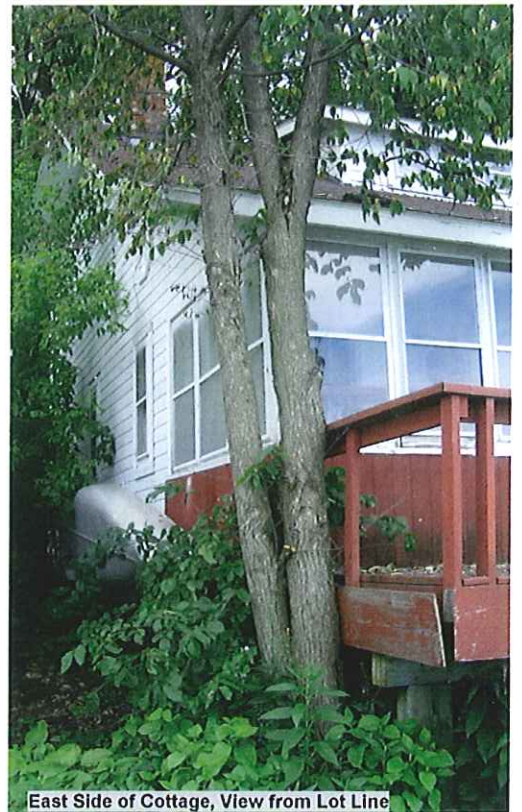
East Side of Cottage, View from Lot Line
