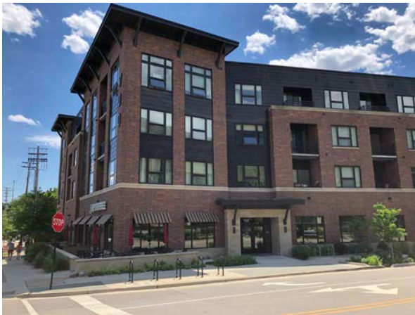
A readily apparent main entrance, materials that change with building articulation, a commercial business emphasized by awnings and outdoor seating, and usable balconies for residential units are all important elements of buildings in the Greater East Towne Area.
