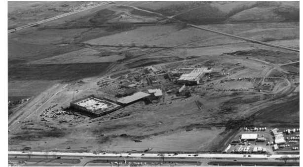
Aerial view of mall construction looking south – 1970
