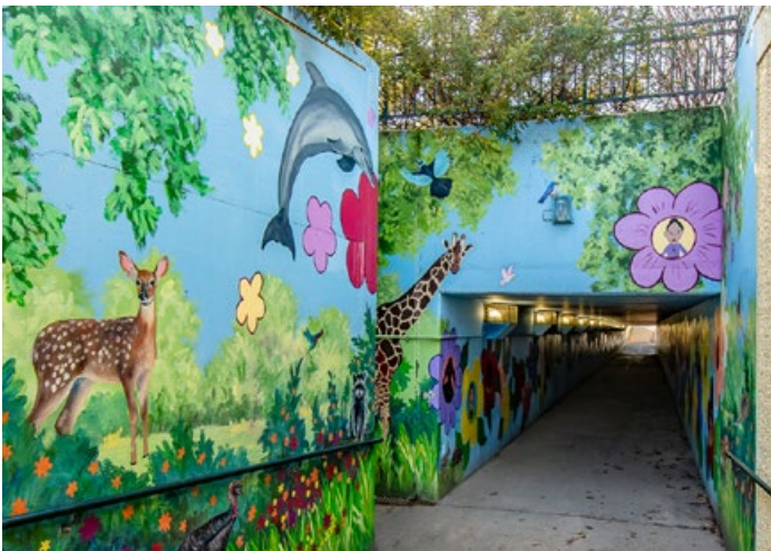
New lighting in the East Washington Avenue pedestrian tunnel at Wright Street
