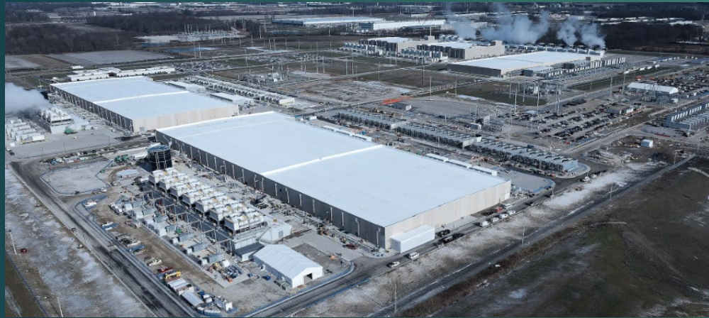
Google Data Center, Council Bluffs IA ( datacenters.google )
