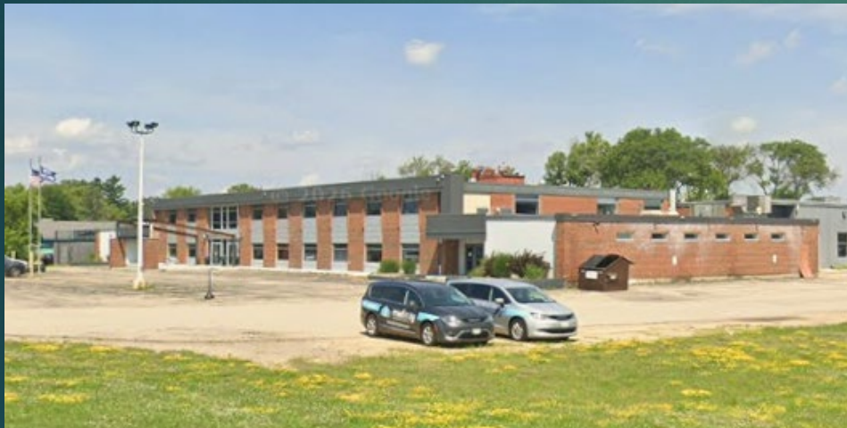
Data Center, 4916 East Broadway, Madison WI
