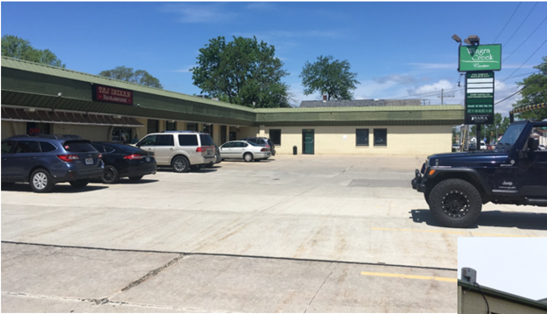
Exterior from Southeast
