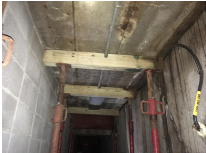
Lower level former office space with temporary shoring posts. Rust staining and spalled concrete visible.
