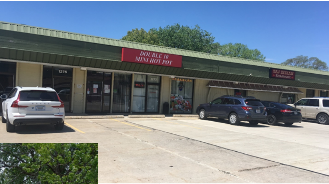
Exterior looking West
