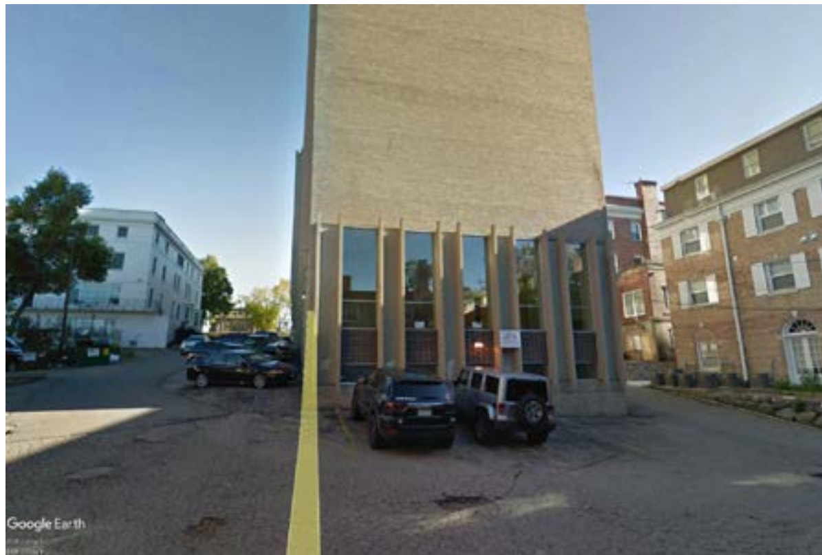
EXISTING SITE, LOOKING SOUTH
