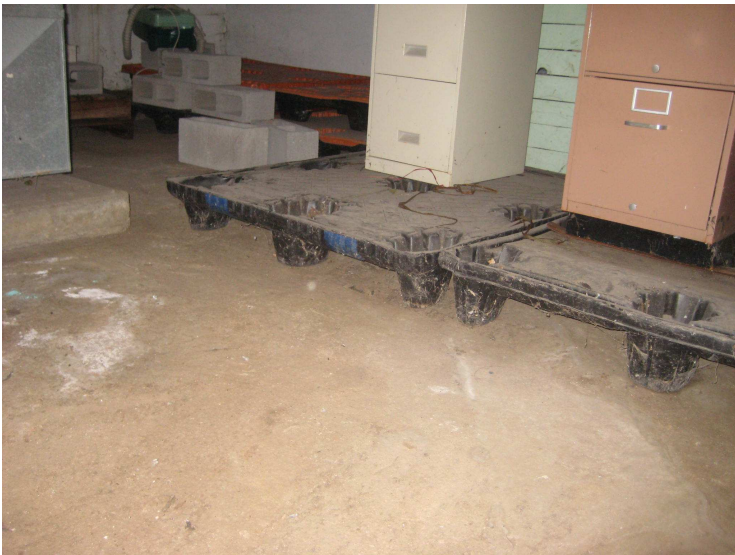
ELEVATED STORAGE DUE TO STANDING WATER
