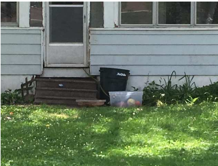
FRONT PORCH STAIR ACCESS
