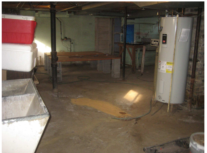
BASEMENT FLOOR/CEILING HEIGHT
