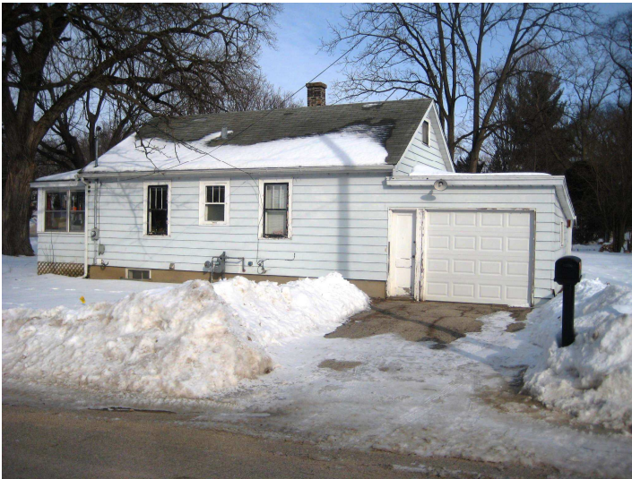
WOODLEY AVENUE/GARAGE VIEW
