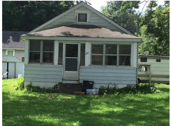
WAUNONA WAY/FRONT PORCH ENTRY VIEW
