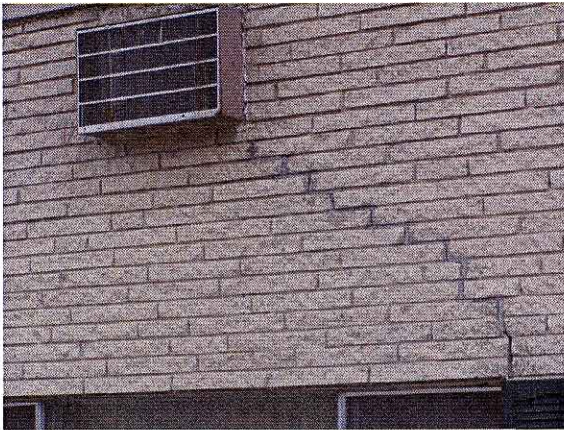
Cracked wall
