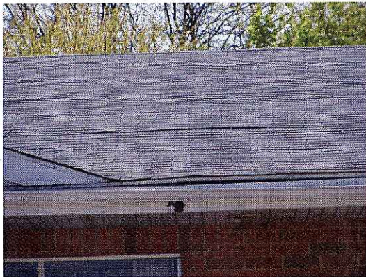
Deteriorating shingles
