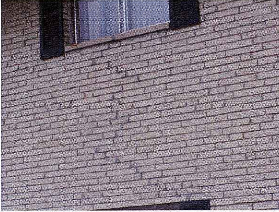
Cracked wall
