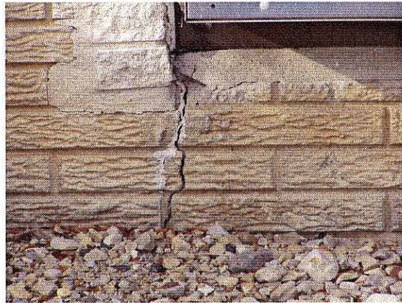
Cracked foundation
