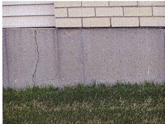
Foundation crack
