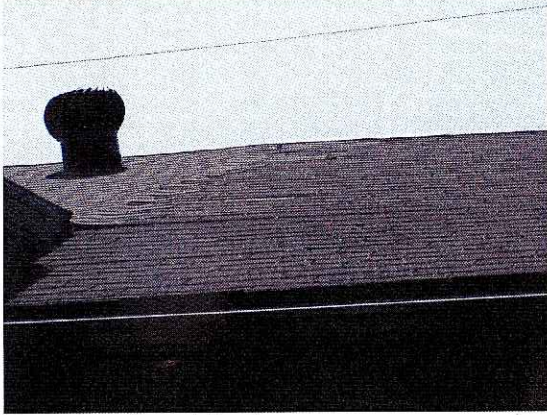
Deteriorating shingles
