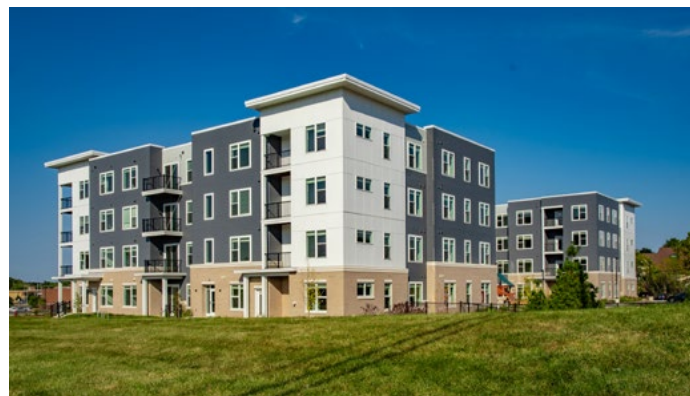
The Derby Apartments added new affordable housing on Atticus Way.
