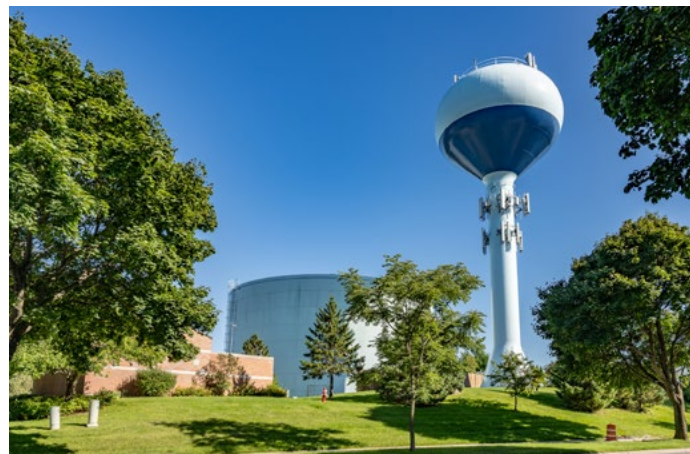
Well 20 serves part of the Southwest Area.
