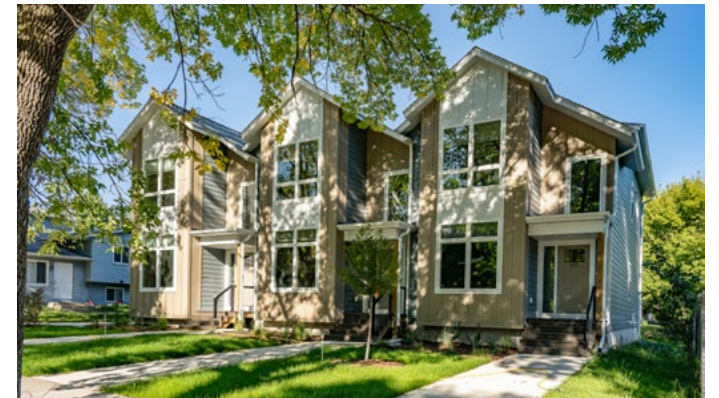
The townhomes on Theresa Terrace were constructed by the Community Development Authority on the site of a dilapidated duplex. It added new Missing Middle housing in the midst of an existing neighborhood.
