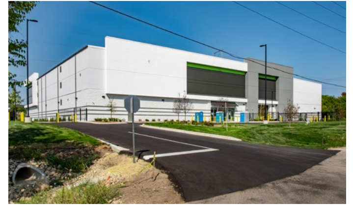
The Extra Space Storage building was recently constructed on a Town of Middleton island at the east end of Seybold Road.
