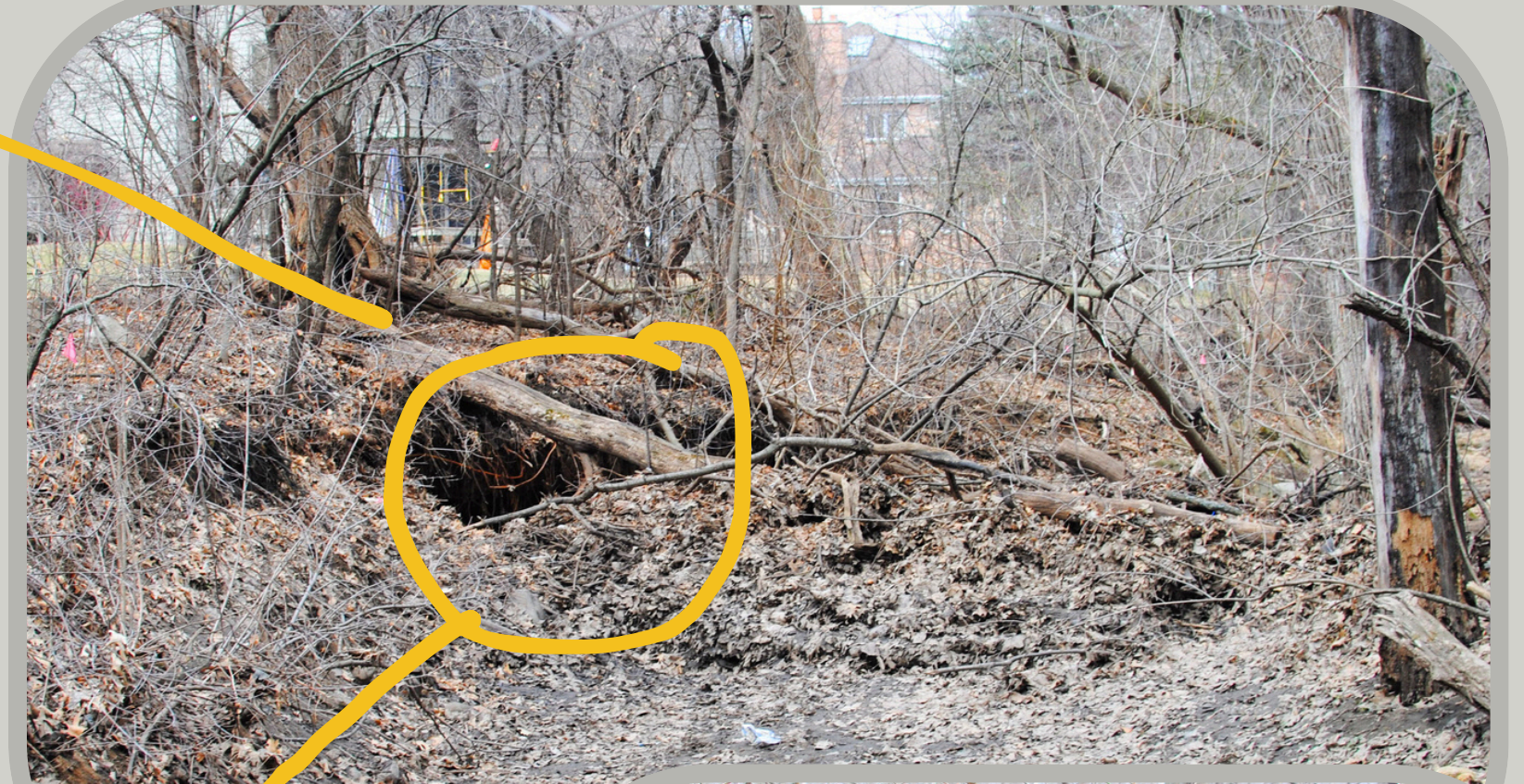
Looking Downstream at blockage
