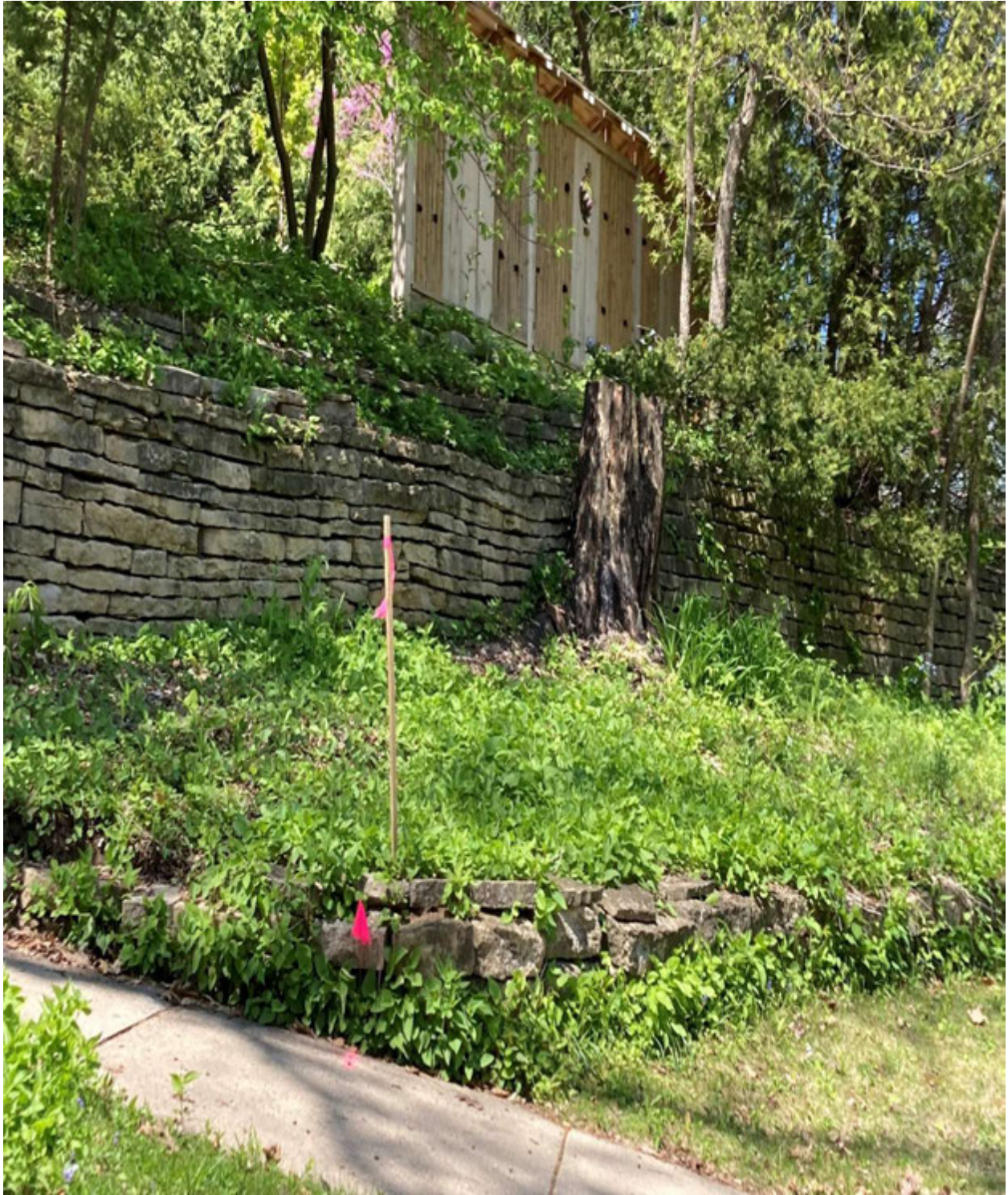
Figure 31 View farther down the stone wall of the Morehouse House. The wall extends about 55 feet, the length of the panhandle between the Morehouse House and proposed Lot 2.
