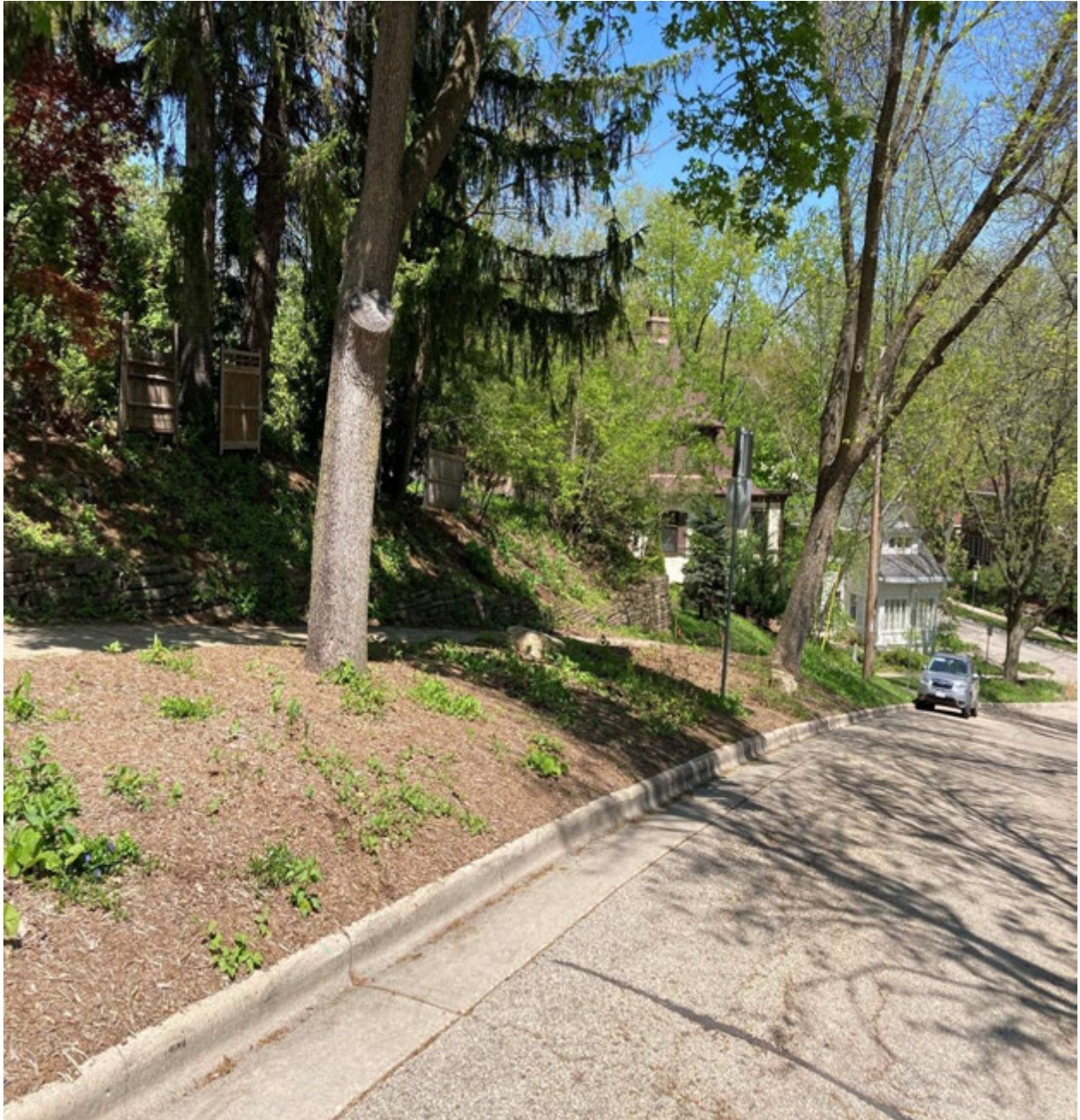
Figure 24 Another view down the hill from Ely Pl to N Spooner St. Note that the fencing on the left and the stone retaining wall in the middle of the photo are property of the Morehouse House. The house at the bottom of the hill, on the flatter lots along N Spooner St., is 202 N Spooner.
