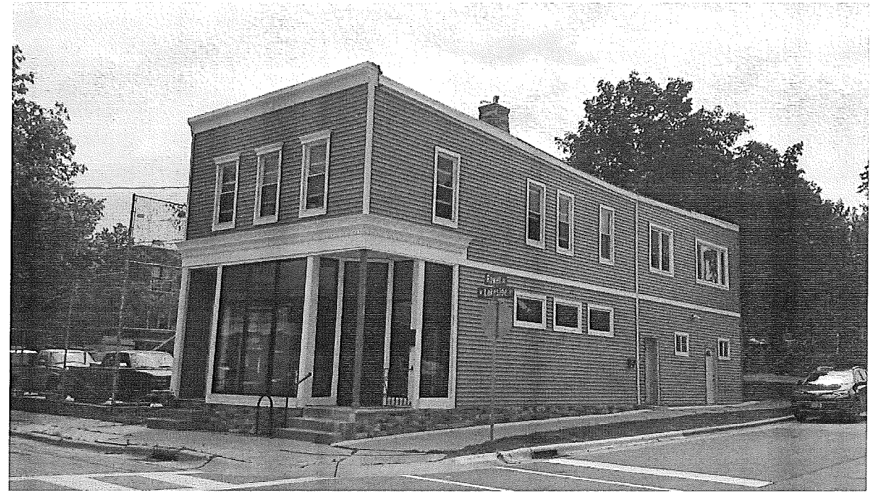
2B Existing Photo - North & West Side of Building 12" = 1'-0"
