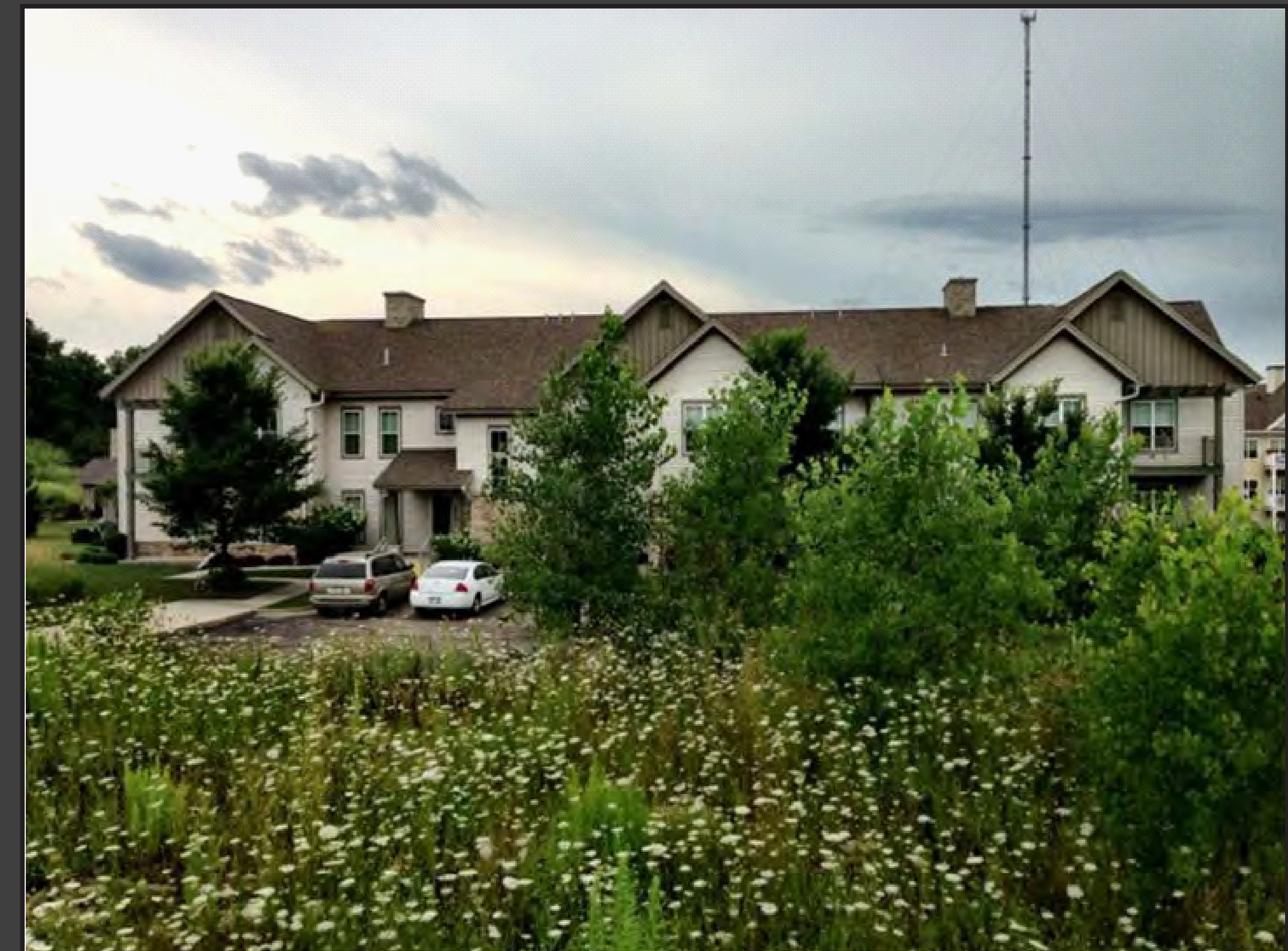
12 UNIT CONDEO, HILLSIDE ESTATES
