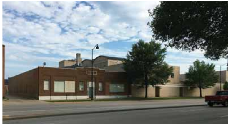
945 East Washington Ave - To be Demolished
