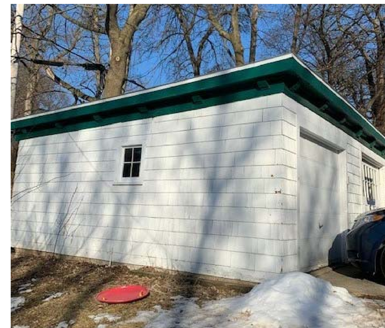
GARAGE SW CORNER
