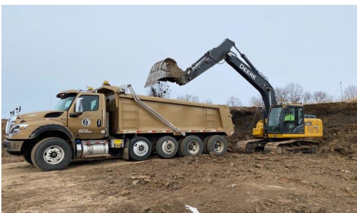
Transporting donated topsoil
