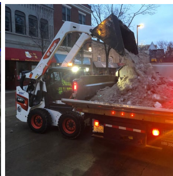
Mall snow removal
