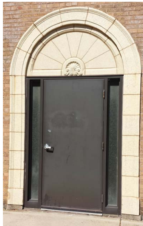
02 EXISTING DOOR to LOWER LEVEL
