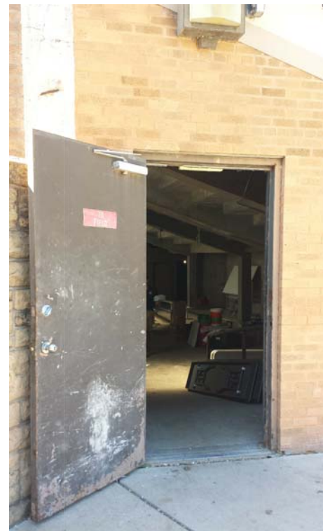
03 EXISTING SERVICE DOOR to LOWER LEVEL
