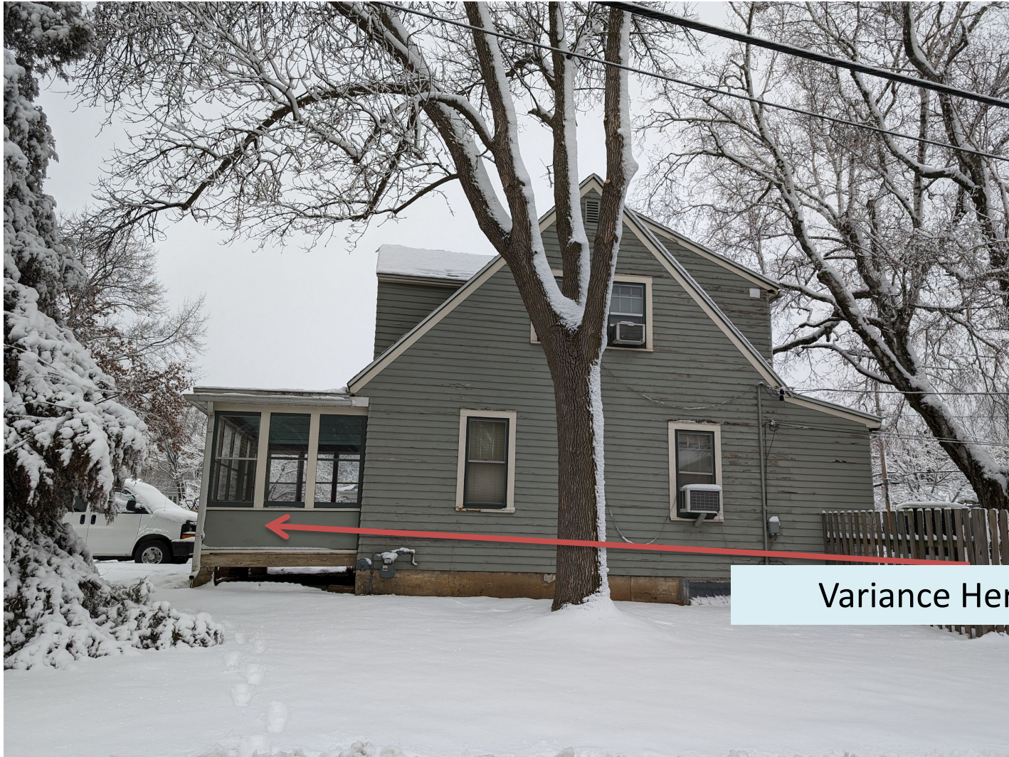
Side East House Elevation – View from Shepard Terrace
