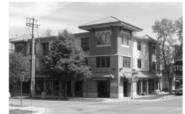
Figure D1: Entrance Orientation
