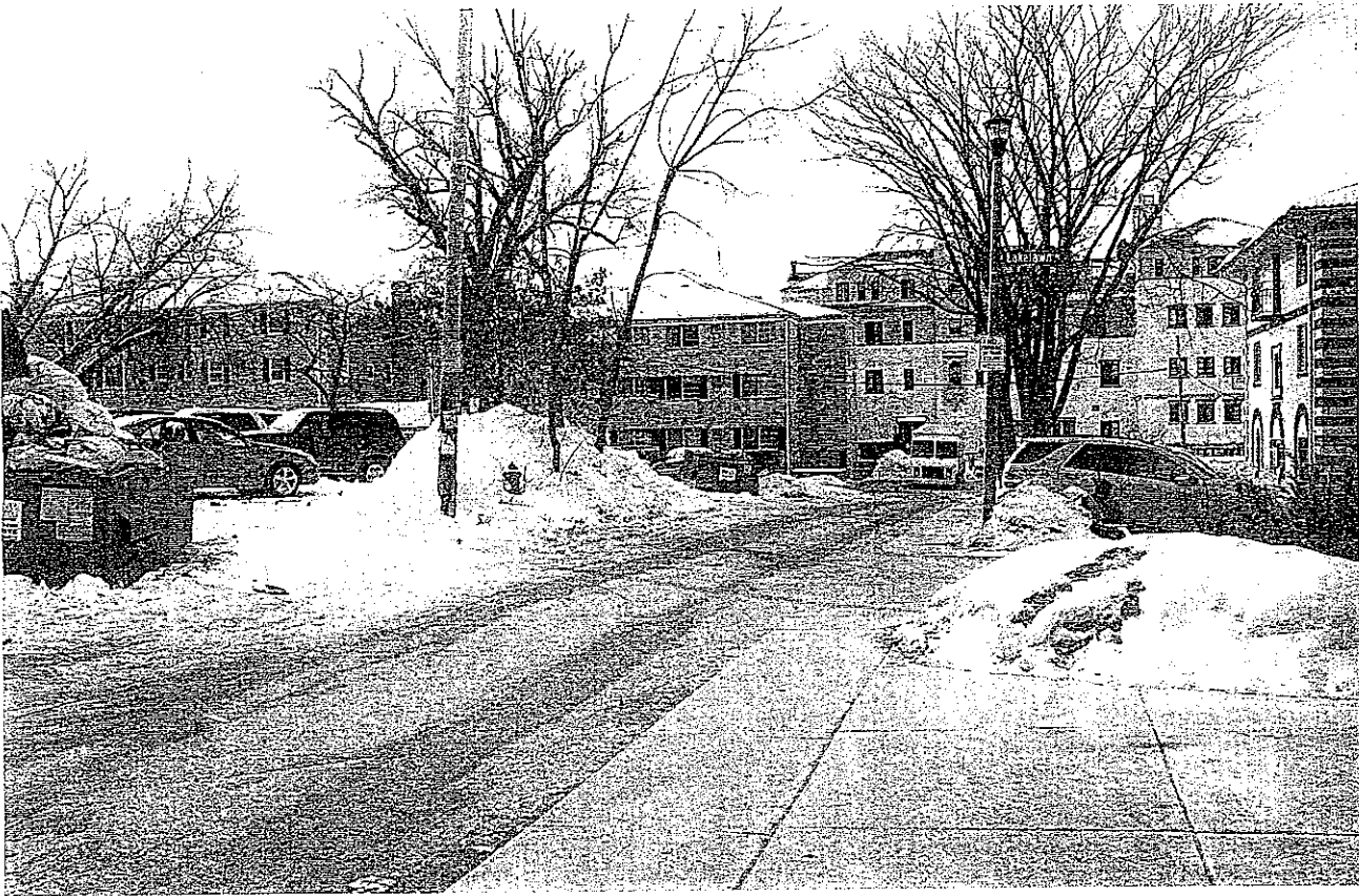
11 - Lakelawn Place (looking Westward)
