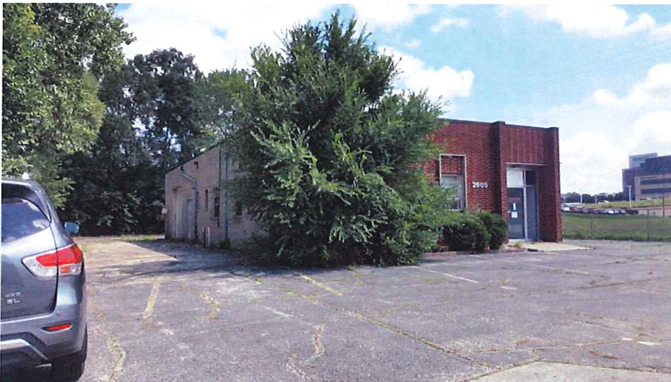
Photo 2: Building exterior, looking southeast.
