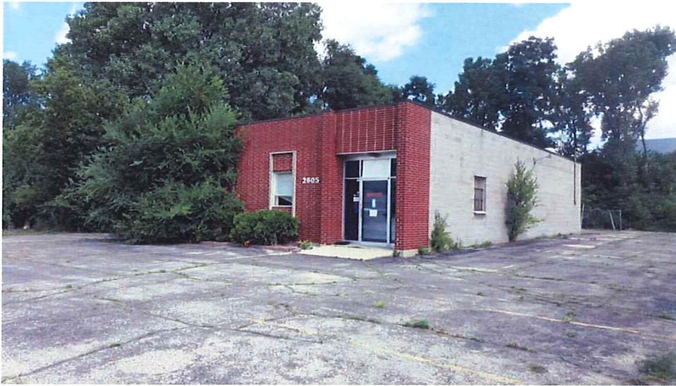
Photo 1: Building exterior, looking northeast.
