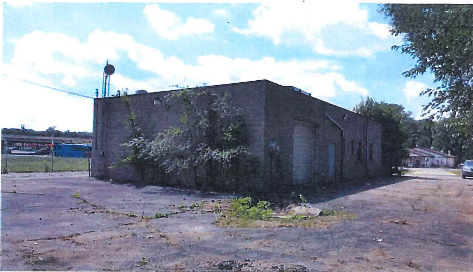
Photo 4: Building exterior, looking southwest.
