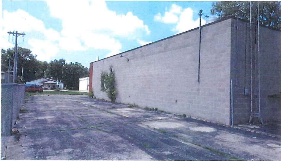
Photo 3: Building exterior, looking northwest.
