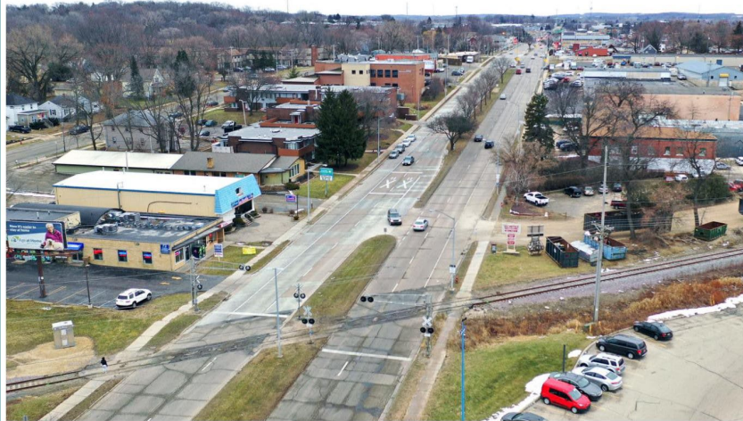
An aerial photo of the South Park Street corridor. Last year, the city purchased property at 1810 S. Park St. for land banking purposes. PHIL BRINKMAN, STATE JOURNAL
