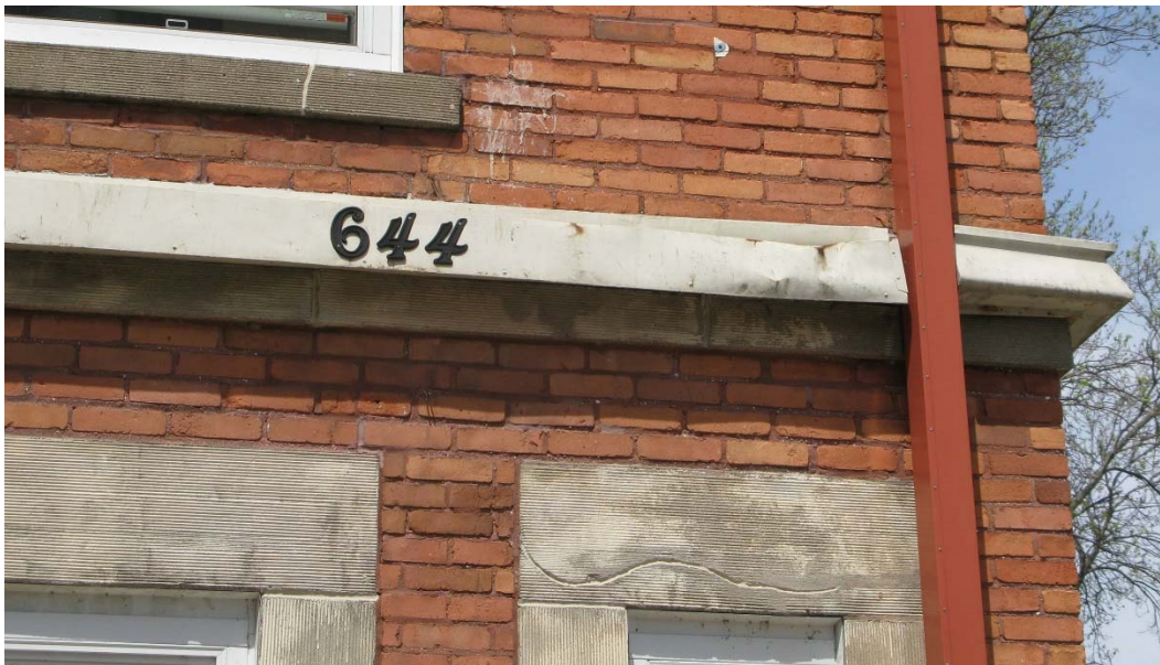
Picture 5977: Damaged non-original metal banding
