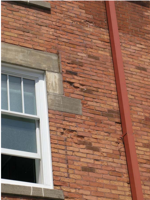
Picture 5961: Typical damaged brick
