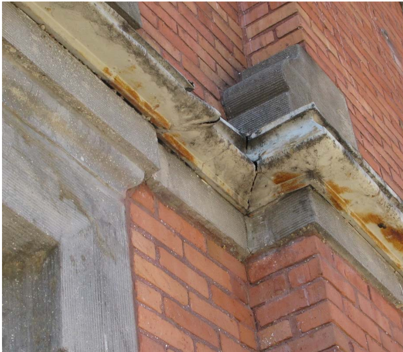
Picture 5913: Damaged original metal banding
