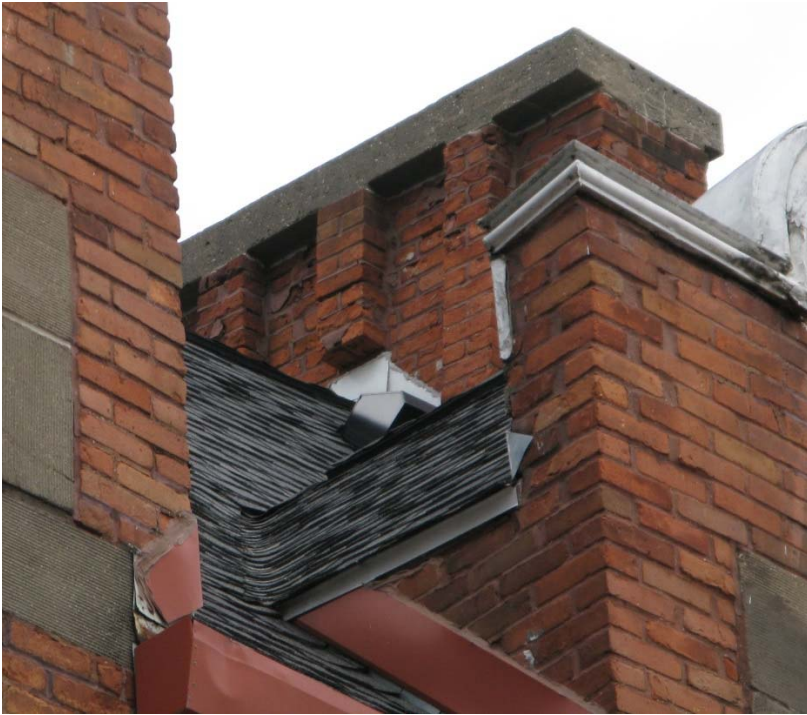
Picture 5956: Chimney repair
