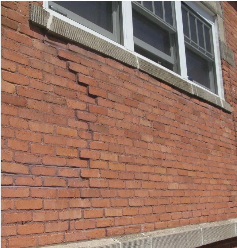
Picture 5960: Crack and bulge
