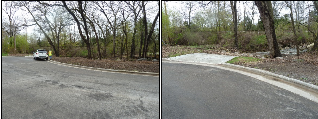
Photos: Improved Street Curb and Gutter. Waite Circle. May 1, 2019.
