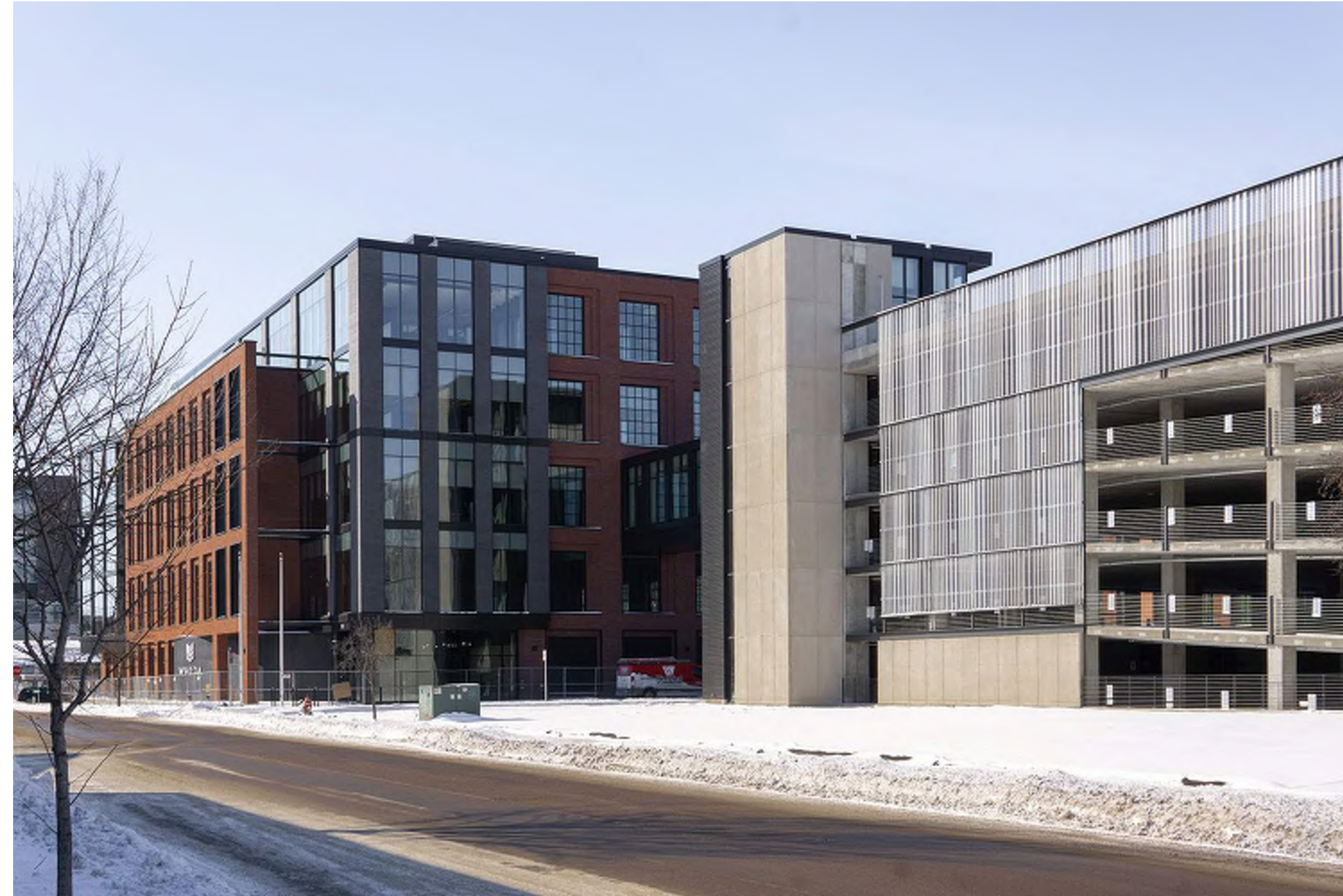
WHEDA Building and Phase 1 Parking Ramp along E. Main St.
