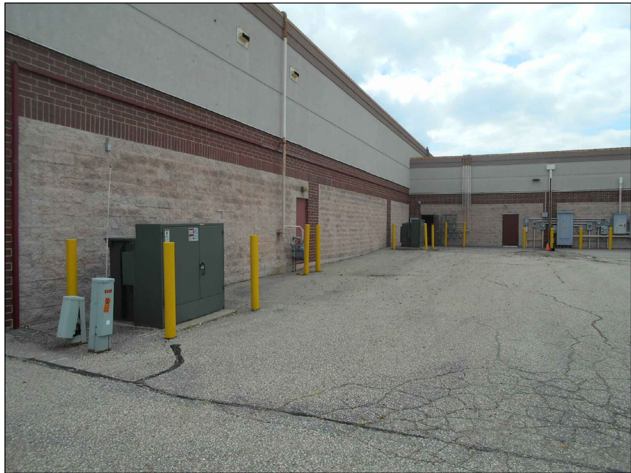
REAR OF EXISTING BUILDING
