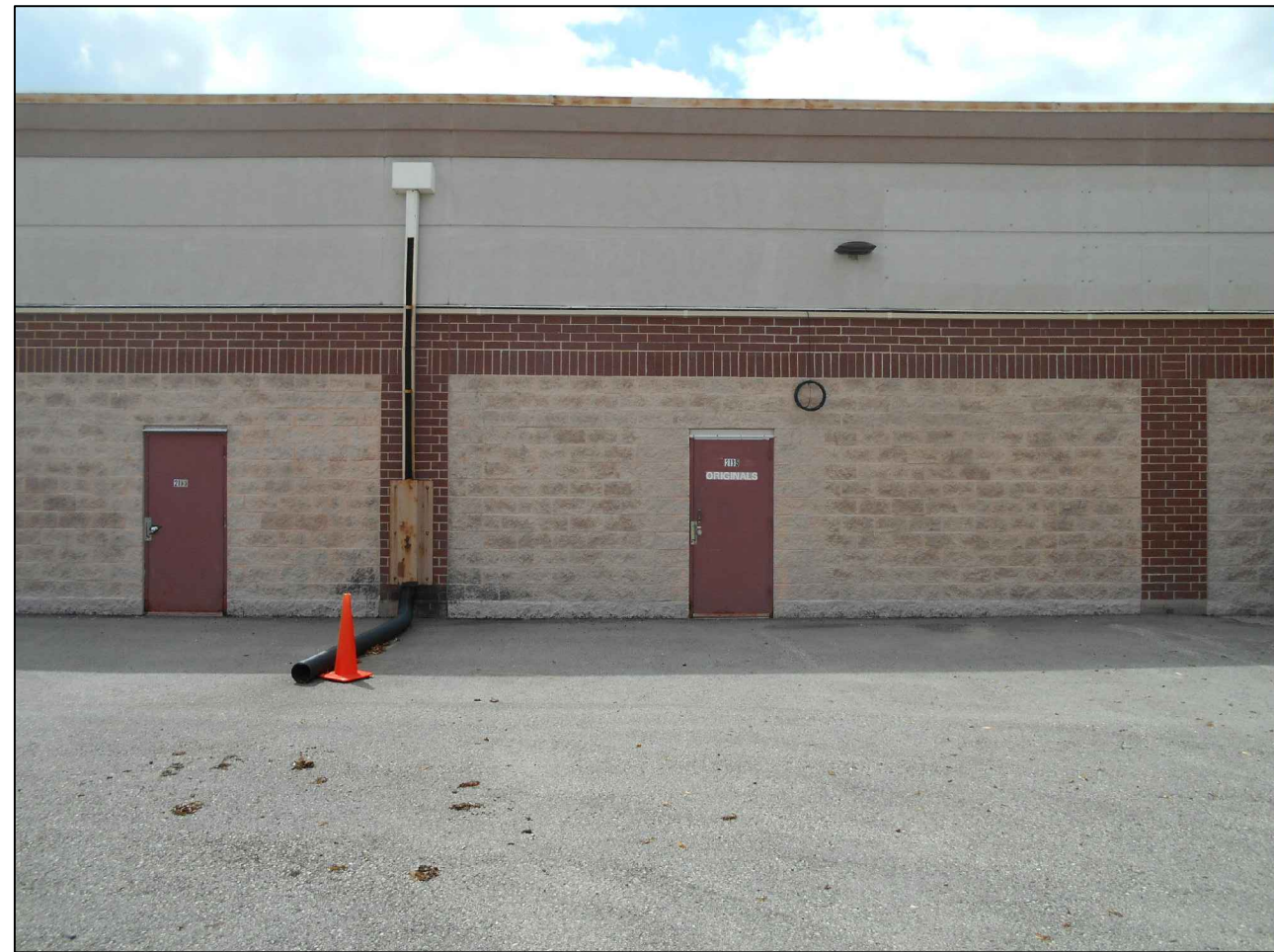
REAR OF EXISTING BUILDING
