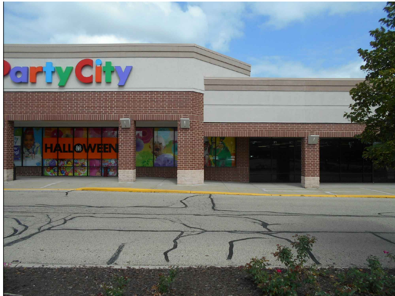
EXISTING CANOPY: LOCATION OF FUTURE ROSS
