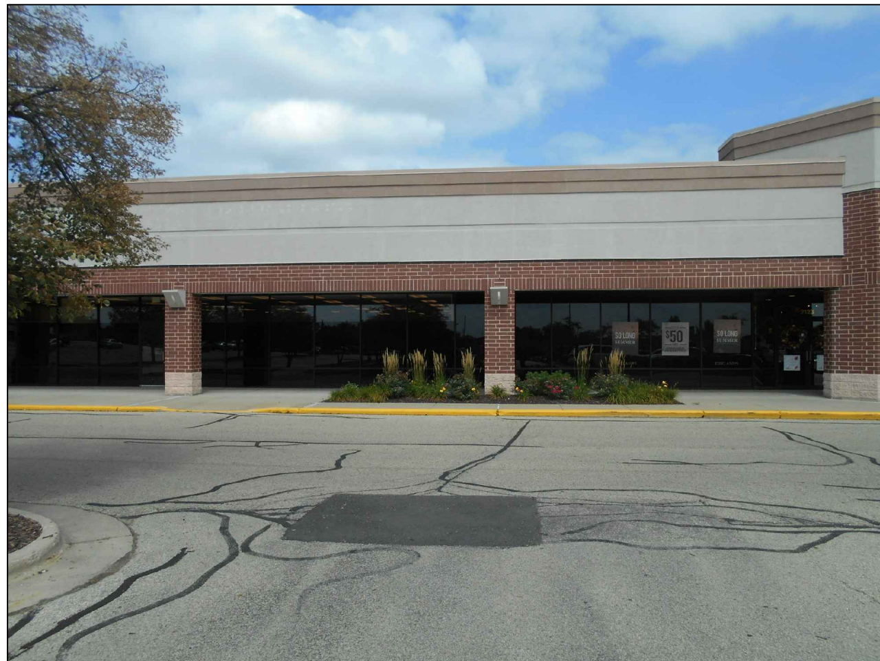
EXISTING CANOPY: LOCATION OF FUTURE ROSS
