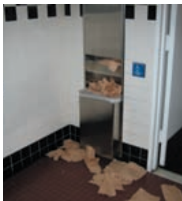
Trash overflow in the Portland Building's men's restroom.
