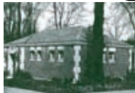
1950s Modernization of existing public restrooms.
