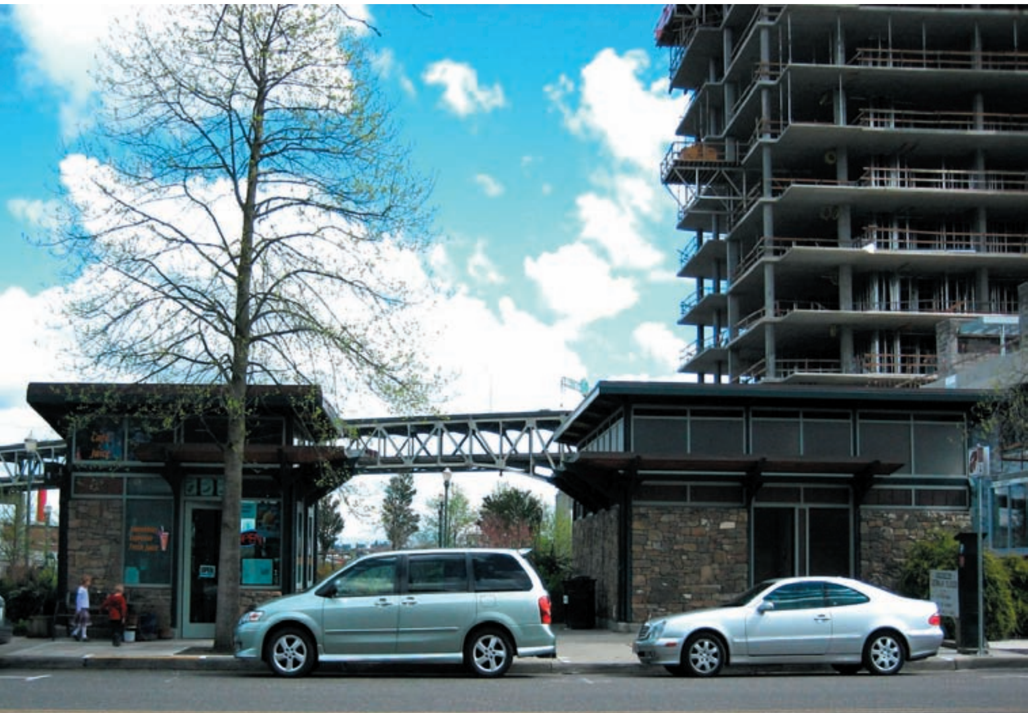
A cafe building adjoins this public restroom at RiverPlace in Portland, OR
