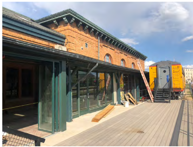
View of the Boardwalk/Deck
